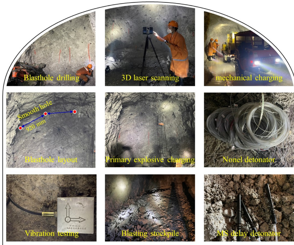
Fig. 3. Blasting operation and field measurement of the test roadway.
