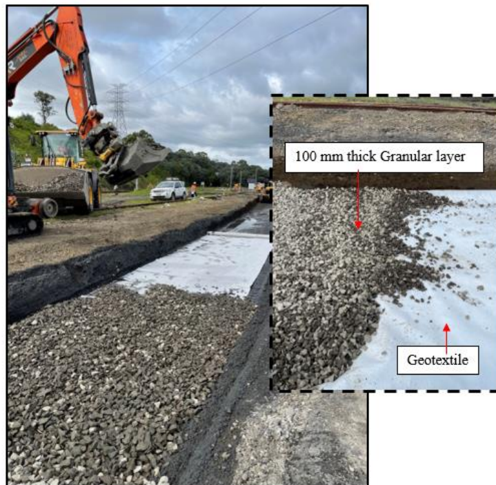
Figure 10. 5: Drainage layer at subgrade level
