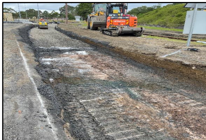
Figure 10. 7: Subgrade soil at Instrumented control section
