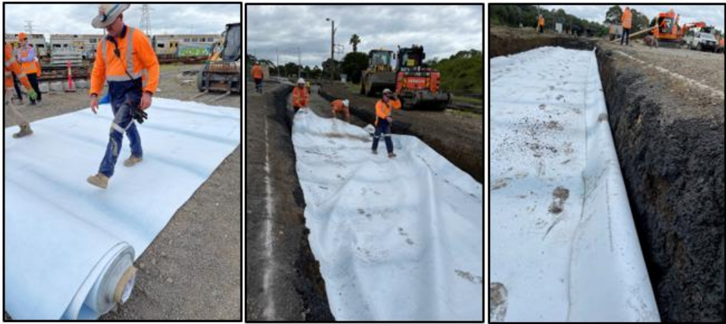
Figure 10. 8: Installation of Terram Hydrotex on subgrade soil – Geocomposite G1
