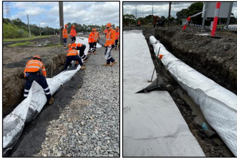
Figure 10. 6: Cess drain construction – 300 mm diameter ag-pipe installation
