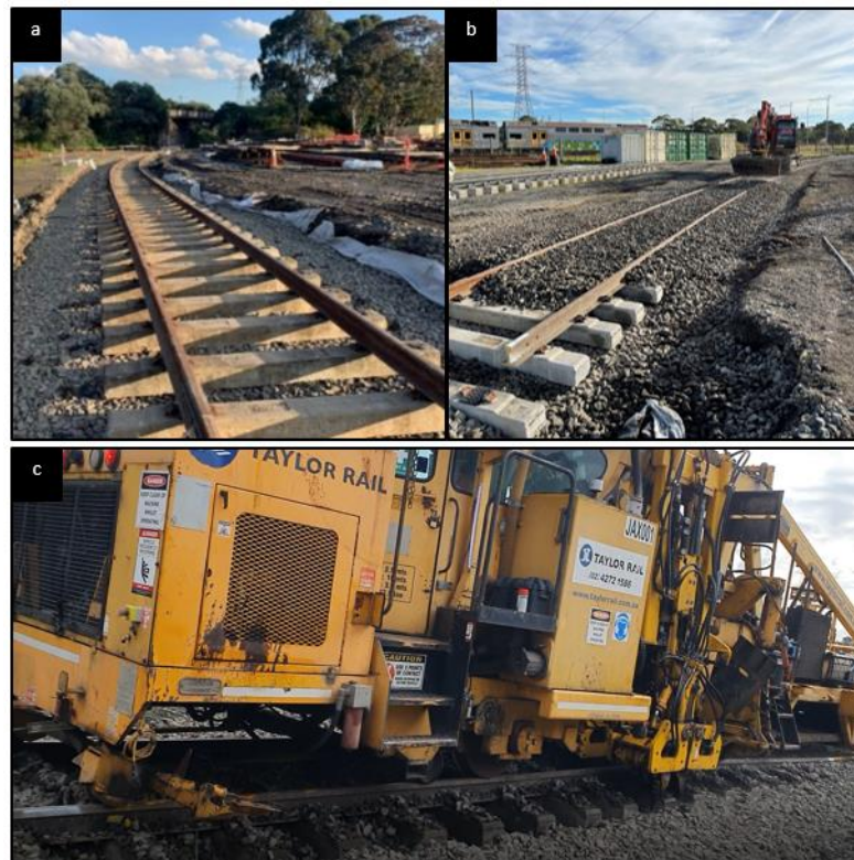
Figure 10.21: (a) Pouring ballast on the instrumentation units, and (b) compaction of 150 mm thick ballast layer
