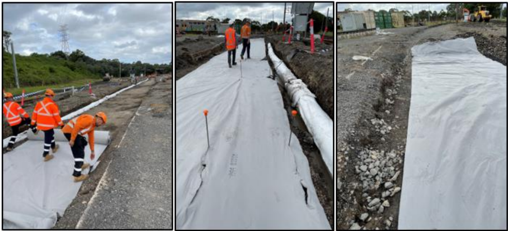
Figure 10. 9: Installation of Bidim A44 on compacted capping layer
