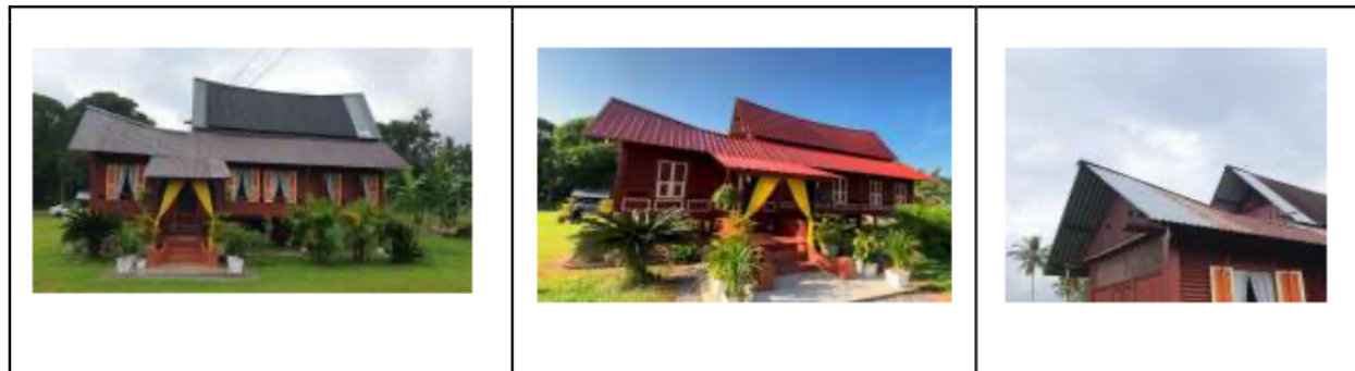
Fig. 10: The roof forms an overhang with slightly upward curves ( lentik ).
