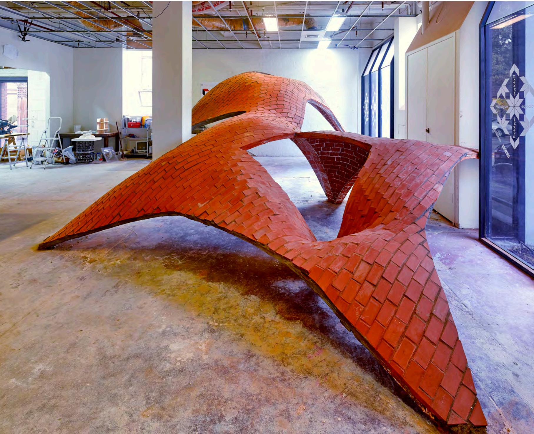
Fig. 1: MADA vault, Melbourne, Australia, 2013. (Photo: Peter Bennetts.)
