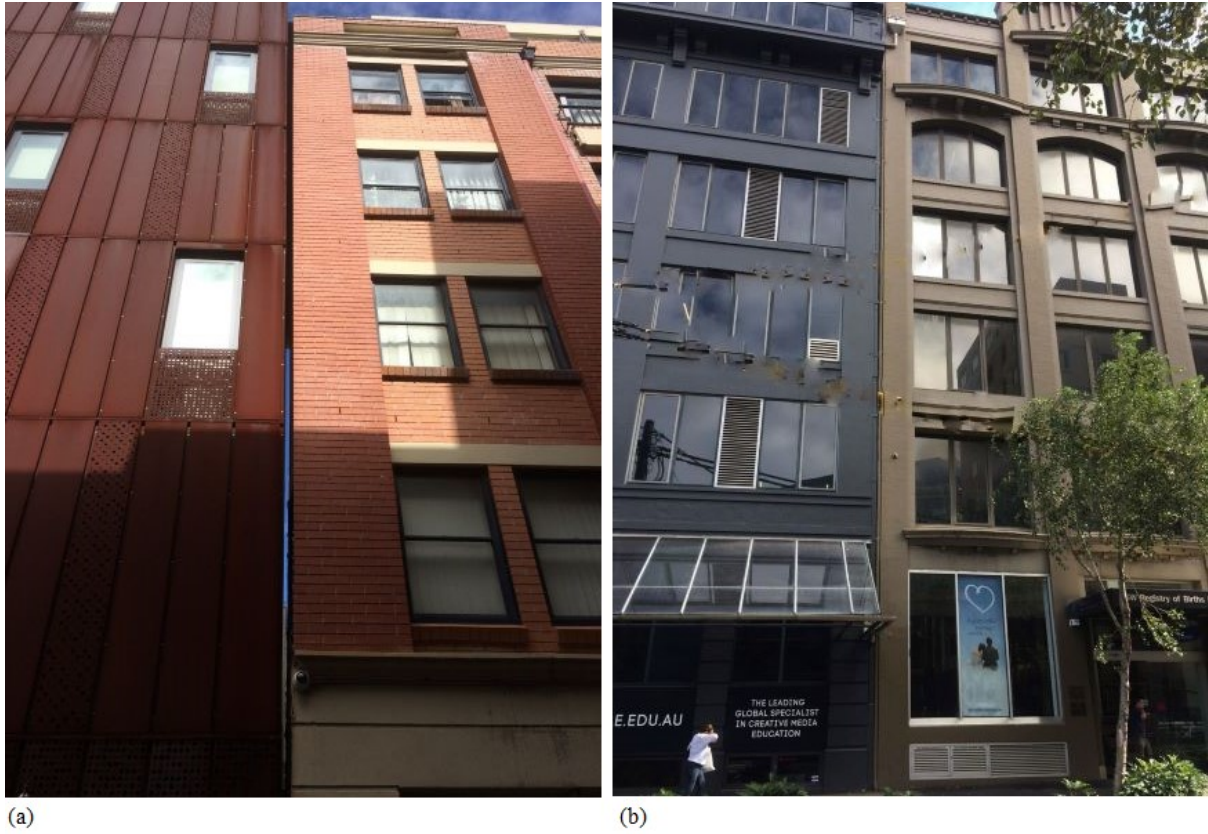
Fig. 1 Case of neighbouring buildings in Sydney, Australia (a) with separation gap; (b) with zero separation gap (image by Yazan Jaradat)
