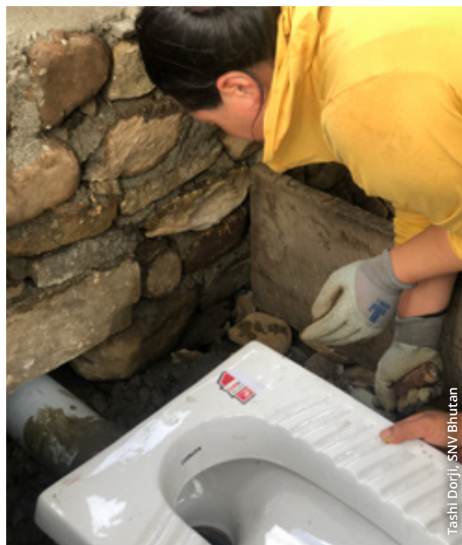
Toilet construction, Bhutan.
