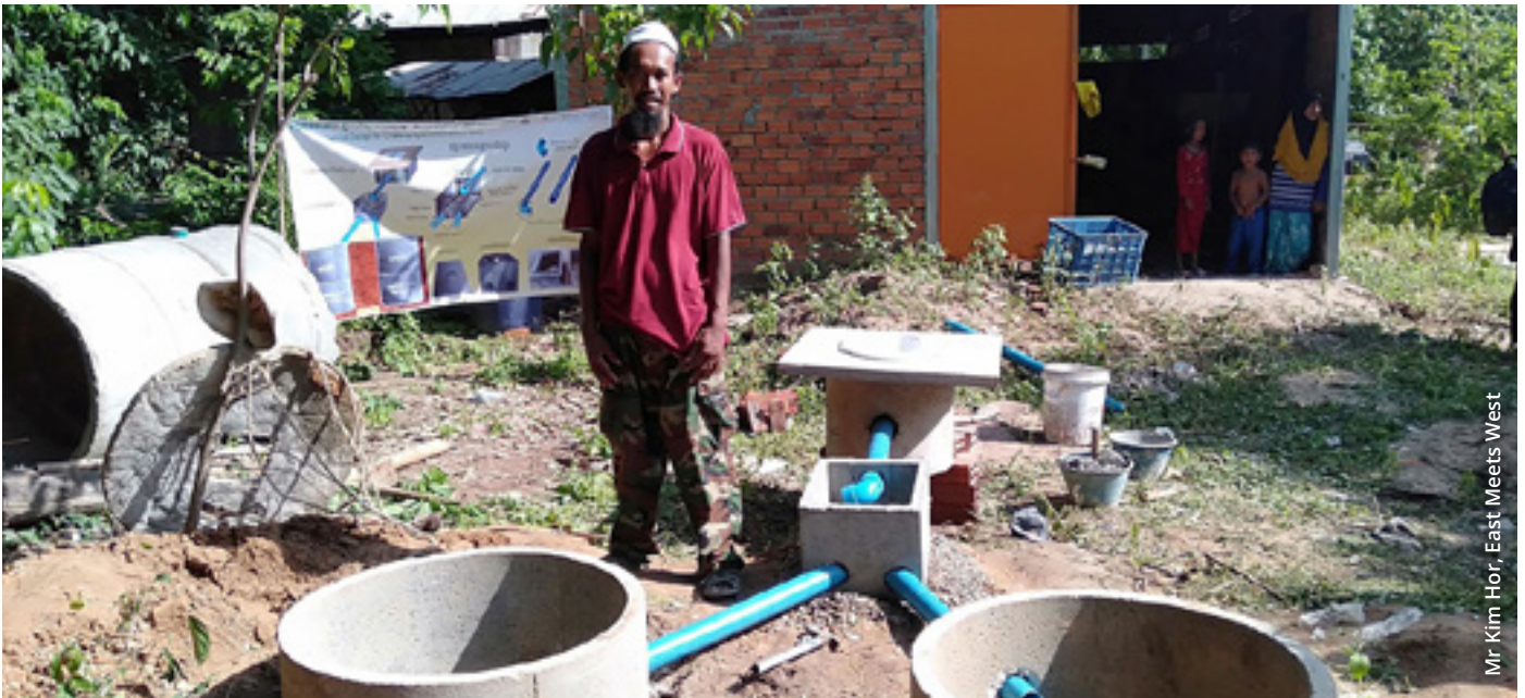
Training of FSM onsite treatment using twin pit household latrine, Kratie province, Cambodia.
