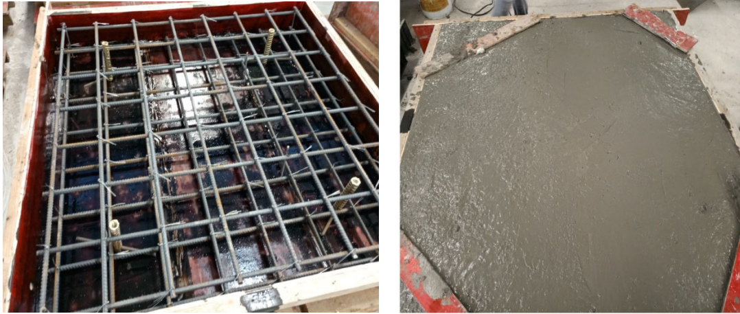
(a) Fabrication of reinforcement
