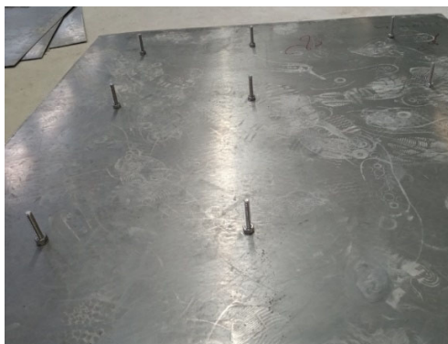
(a) Fixing the stainless-steel bolt connectors
