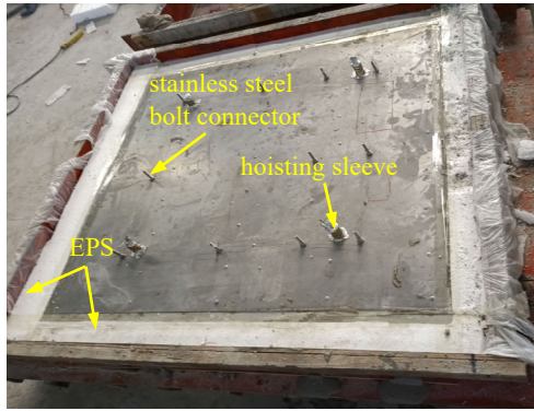
(c) Installation of EPS
