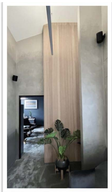
Figure 6.6 Sonos wall speakers Sonos speakers, shown on the northern and southern walls of the waiting room, with sub-woofer placed out of sight in corner
