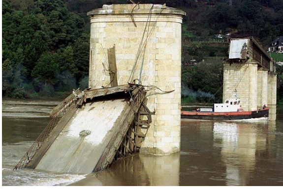
(a) Hintze-Ribeiro Bridge collapse
