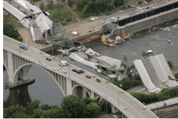
(b) Minnesota River Bridge collapse
