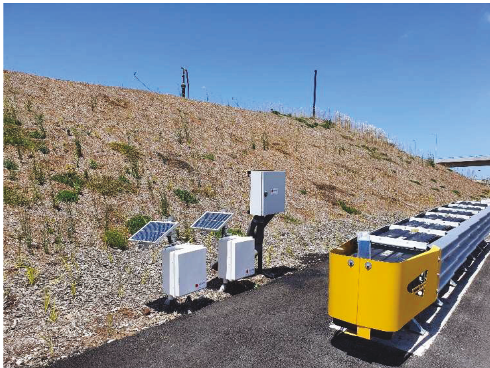
Figure 7.11 After embankment construction
