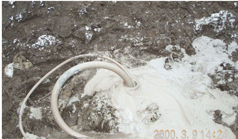
Figure 2.20 Fly ash mixture with the injection hose and hydraulic hose (Fatahi, 2012)
