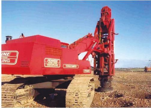
Figure 2.12 Rapid Impact Compaction rig (after Serridge and Synac, 2006)
