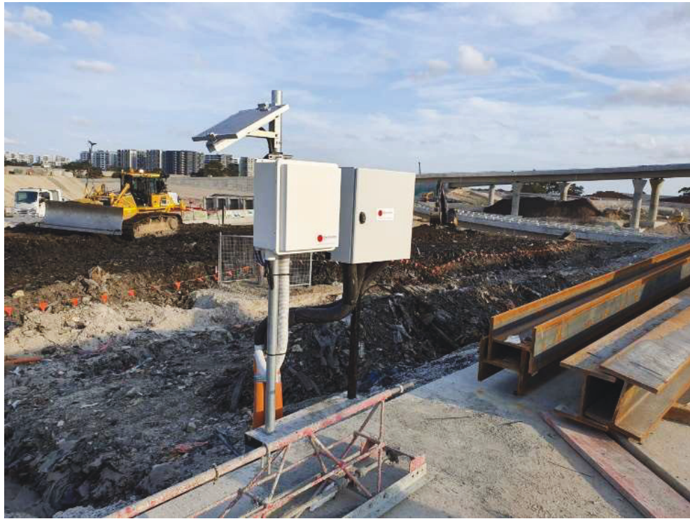
Figure 7.10 Before embankment construction
