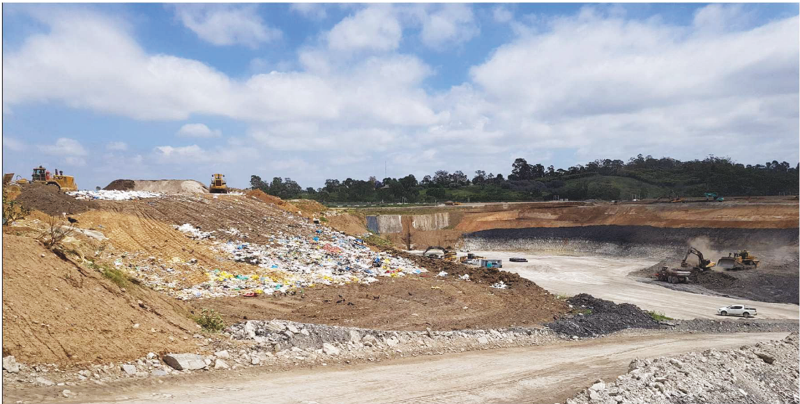
Figure 1.1 Landfill in Western Sydney (photo taken by the Author)
