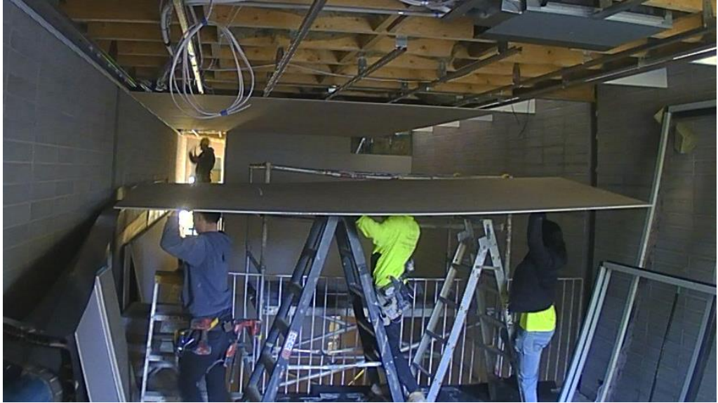
Figure 4.4: Movement of the drywall sheets
