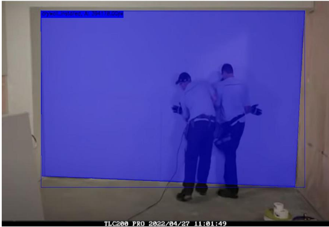
Figure 5.23: Indoor partition wall is fully installed
