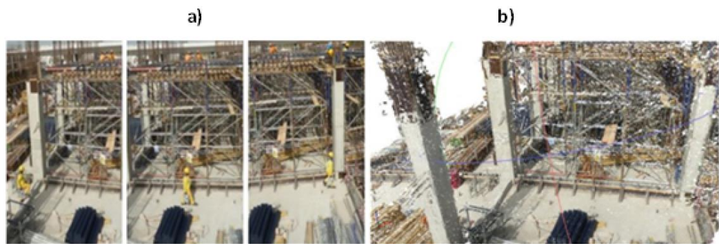
Figure 2.6: A construction site a) 2D image; b) 3D photogrammetric model
