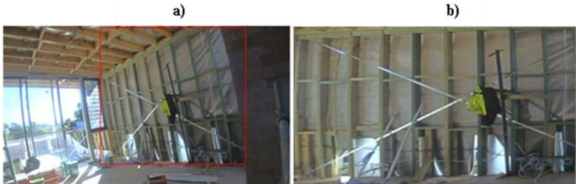
Figure 4.18: Perspective transformation: a) Original image; b) Corrected image
