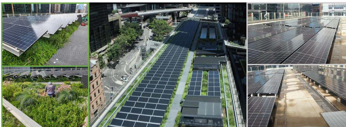
Figure 25. Aerial image of the study site (centre image). Daramu House (bio-solar; left two panels) and International House (conventional solar; right two panels). Sister buildings were near-identical with the exception of roof surface cover (plant material vs concrete). Plant material covers all regions of below panel areas on the bio-solar roof.
