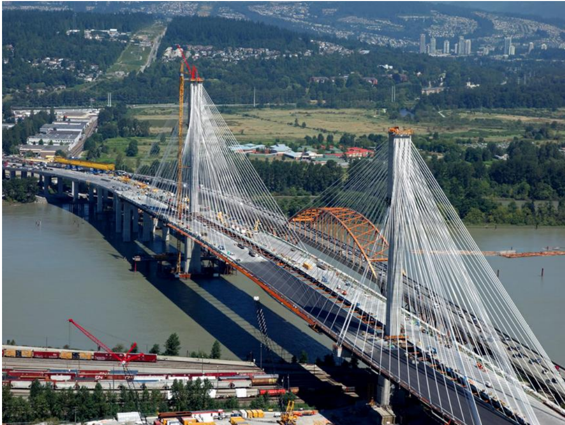
Figure 4.2 The Port Mann Bridge in British Columbia
