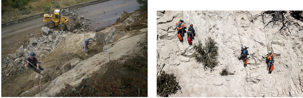
FIGURE 1.1: Abseiling workers performing manual rock-scaling operations.
