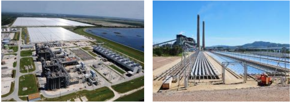
Figure 21: 75 MW e Martin integrated solar combined cycle plant in Florida, USA (left, from NREL [102]) and 9.3 MW th solar integration at Liddell coal fire station in Liddell, Australia (right, from ProTender [103]).
