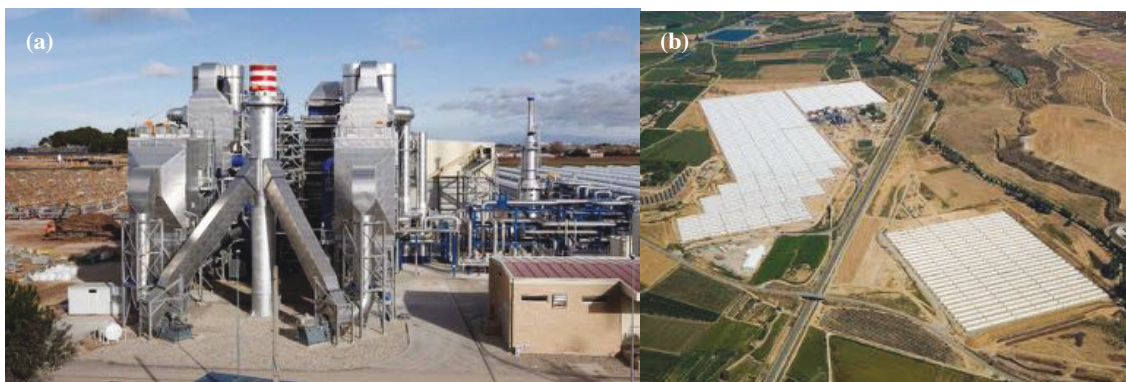
Figure 9: Termosolar Borges plant in Lleida, Spain: (a) bioenergy system and steam cycle, and (b) parabolic trough collector field. Source: Power Technology [31], and Crespo [32].
