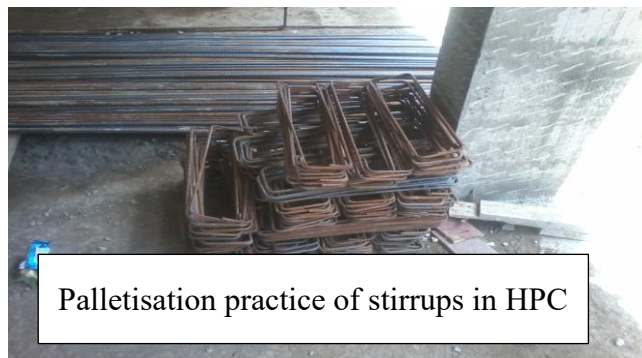
Figure 4.4 Palletisation of stirrups in HPC and APC and wastage of rebars in APC
