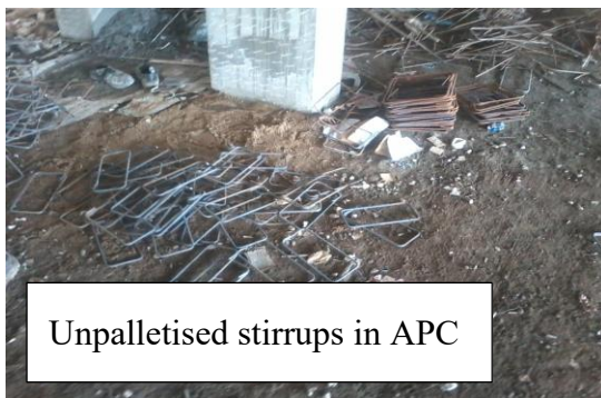
Figure 4.4 Palletisation of stirrups in HPC and APC and wastage of rebars in APC
