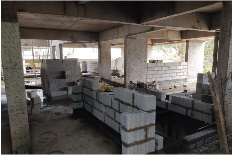
Figure 6.6 Case GREEN showing the ongoing brickwork construction activity
