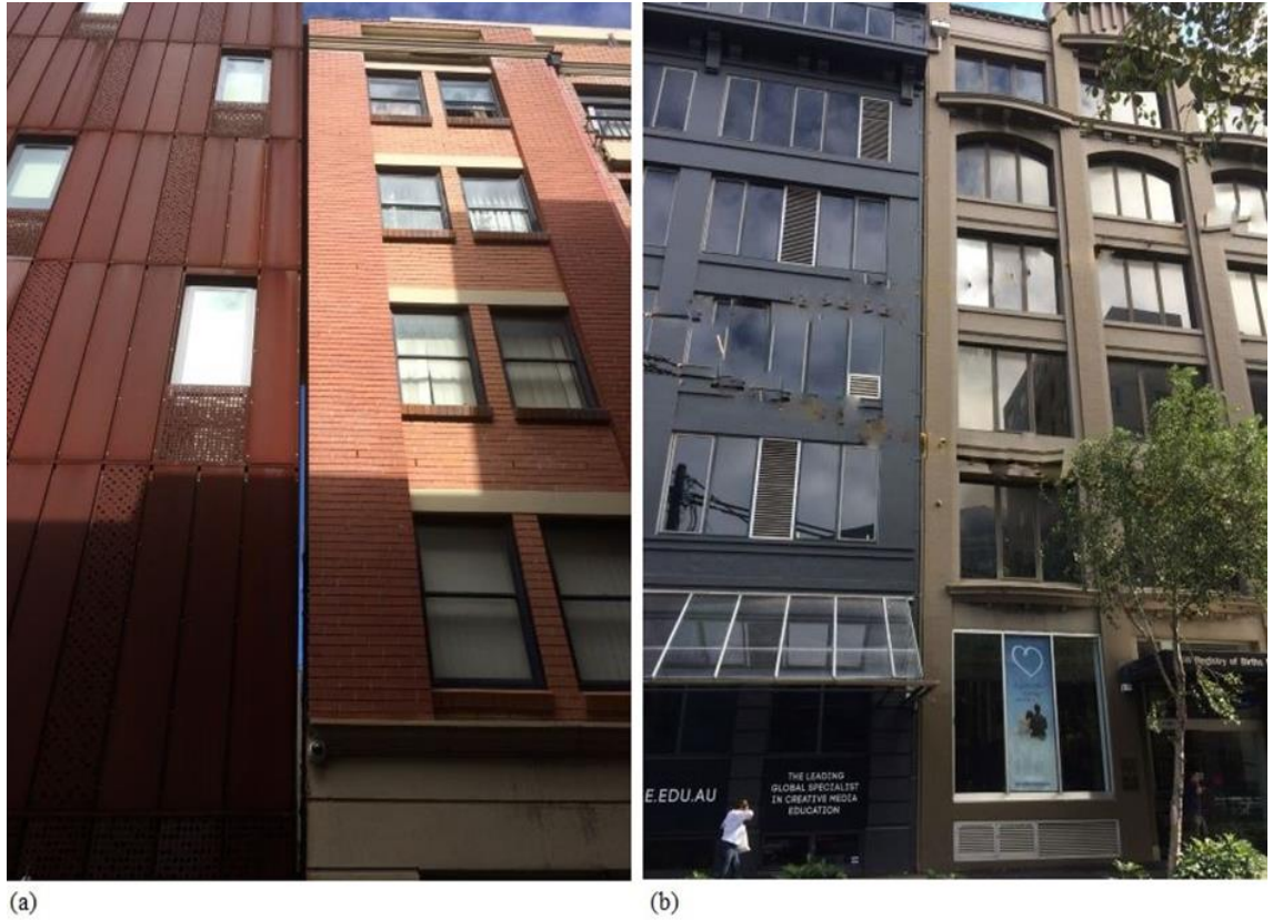
Figure 4.1 Case of neighbouring buildings in Sydney, Australia (a) with separation gap, (b) with zero separation gap (image by Yazan Jaradat)
