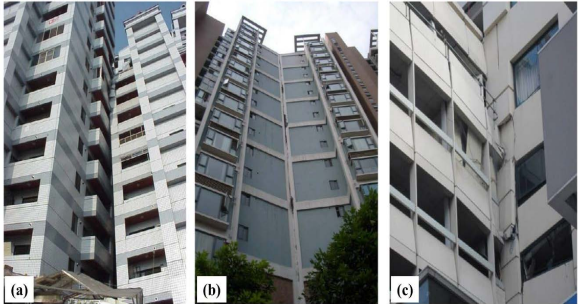
Figure 1.1 Detected pounding damage between adjacent structures: (a) 1999 Taiwan earthquake (b) 2008 Wenchuan earthquake (c) 2011 Christchurch earthquake (Hao 2015).
