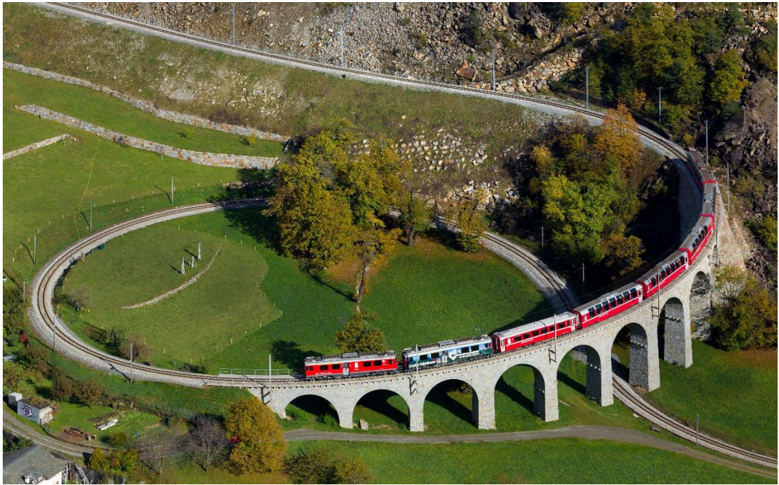
Figure 2.3: Local train crossing the Brusio spiral viaduct, Switzerland (Gubler 2012)
