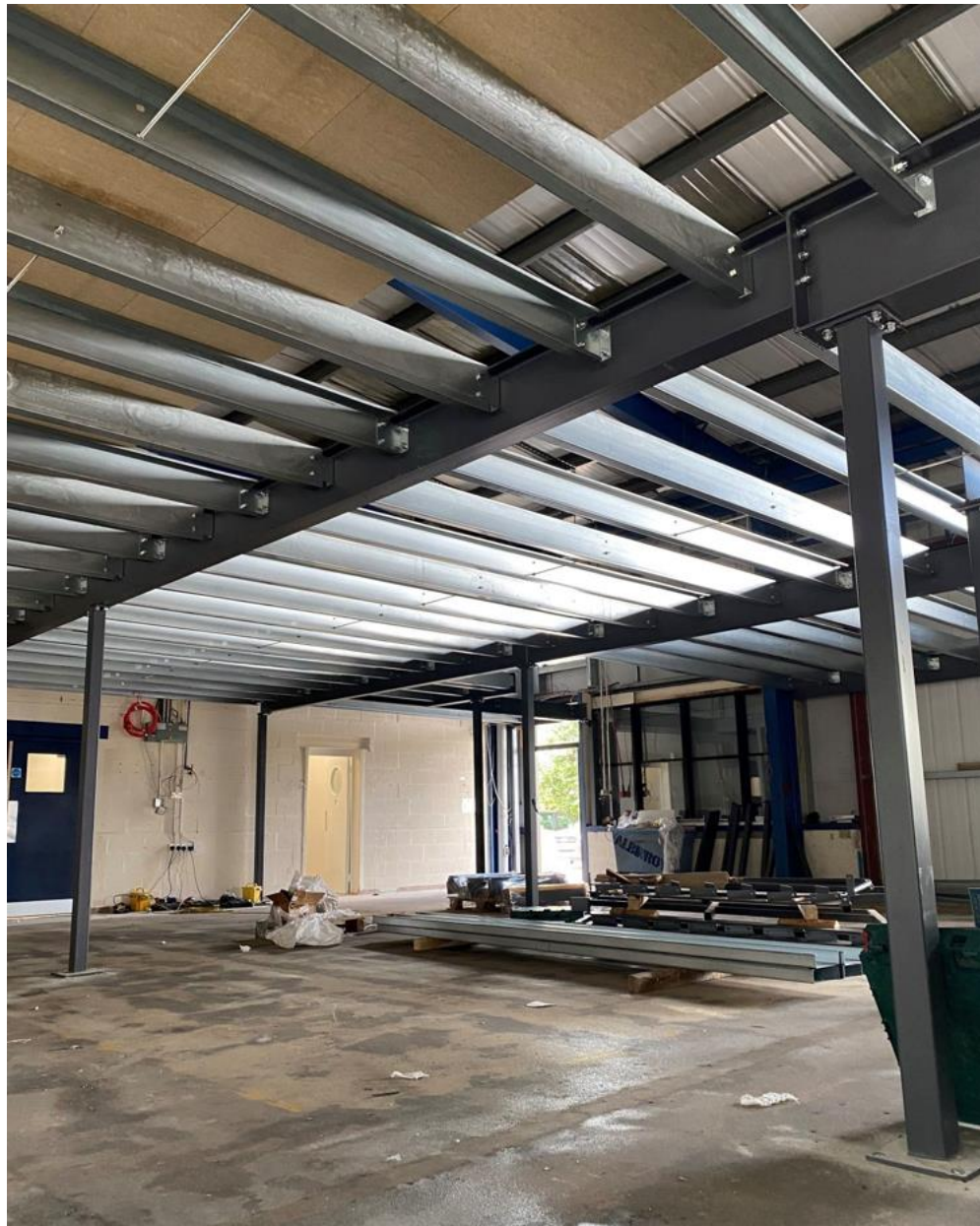
Figure 2.10: Construction of a mezzanine floor using CFS joist and timber floorboard sheathing (Ayrshire Metals Ltd UK, 2022 )
