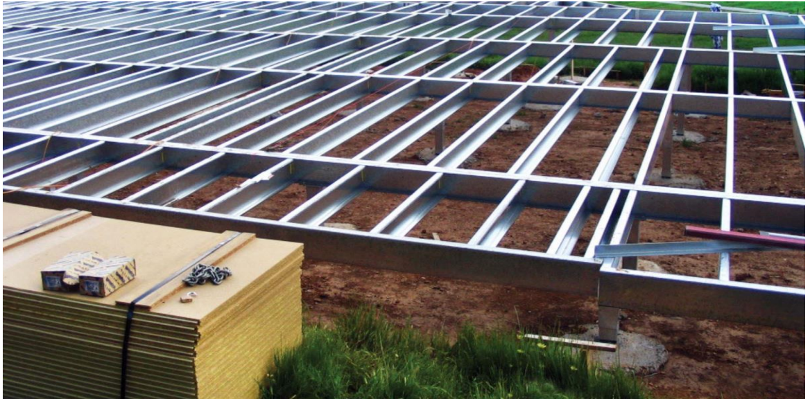
Figure 1.2: A typical domestic raised floor system using cold-formed steel joists (Stratco Australia, 2019).
