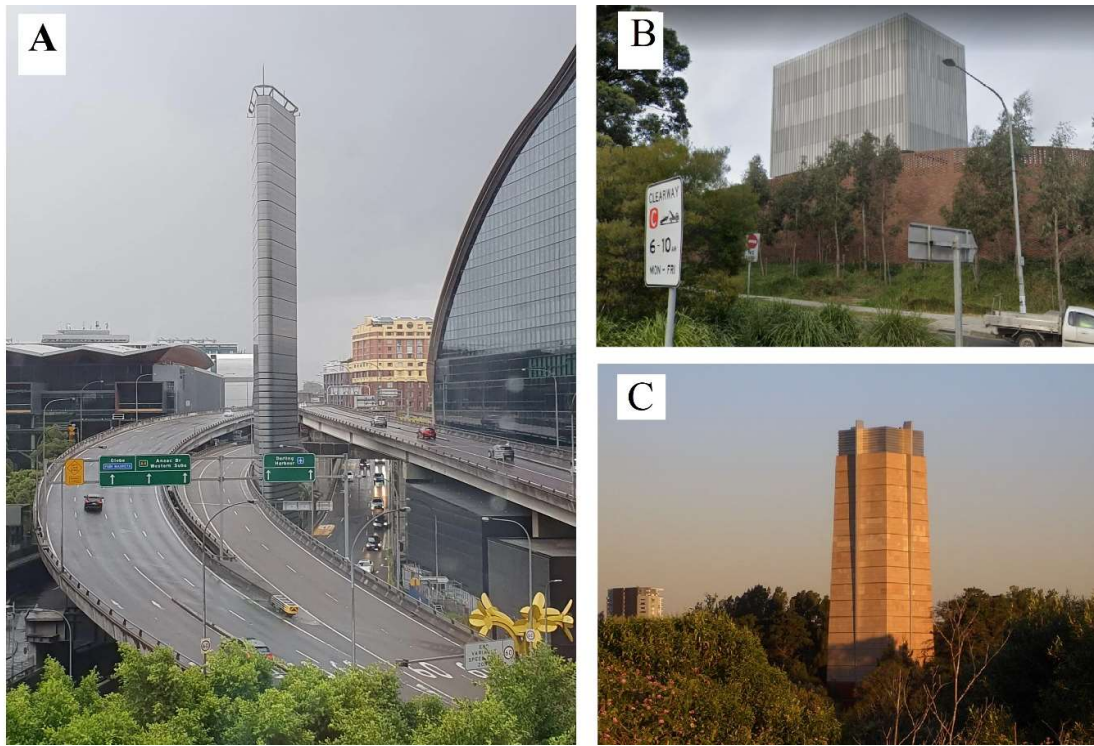
Figure 1. Ventilation stacks for existing road tunnels across Sydney Australia. A.) Cross City Tunnel, B.) M4 Extension, C.) M5 East.
