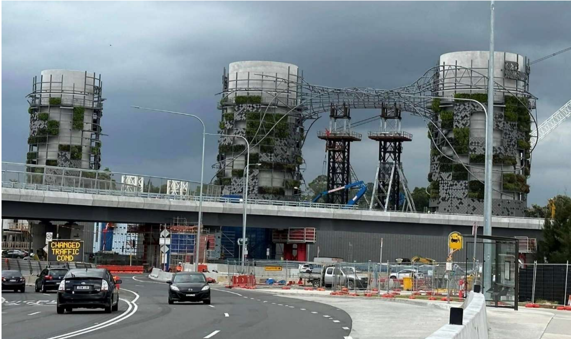
Figure 3. Tunnel ventilation stacks with completed installation of all the green wall modules. Ventilation stack 1 is furthest to the right, followed by Ventilation Stack 2 in the middle, and Ventilation Stack 3 on the left.
