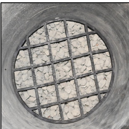
Placing rubber grid at ballast capping interface
