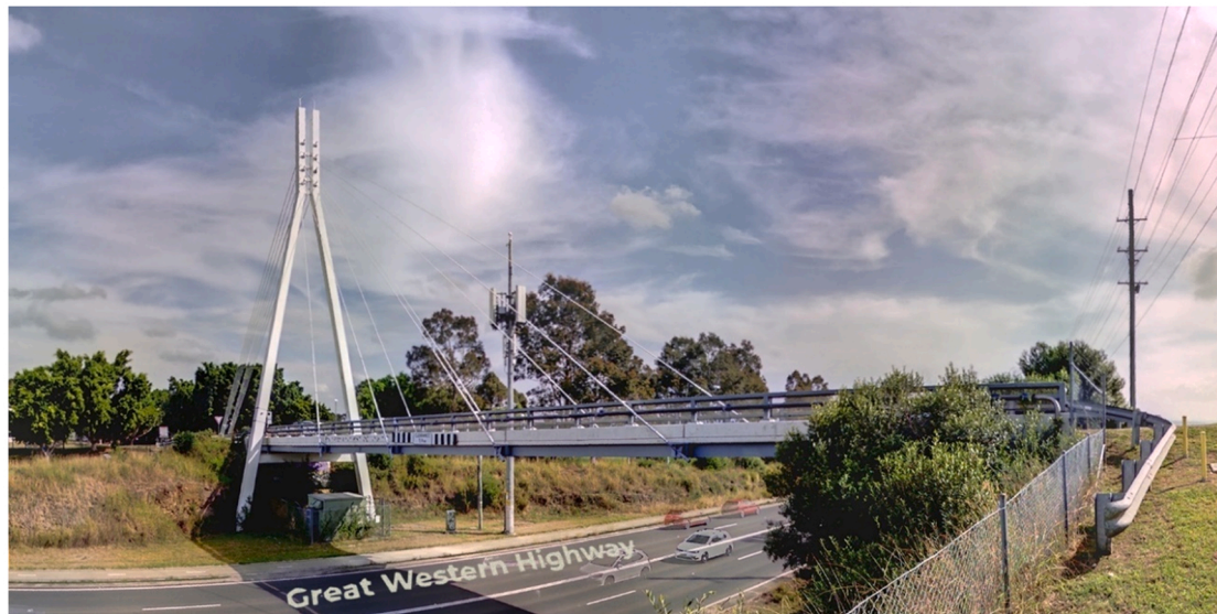
(b) Bridge view in 2021
