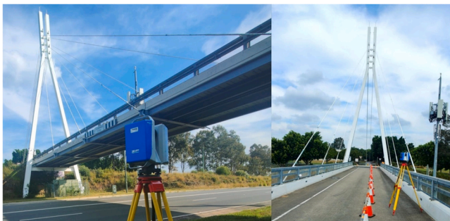
Fig. 4. Werrington bridge data acquisition via TLS.
