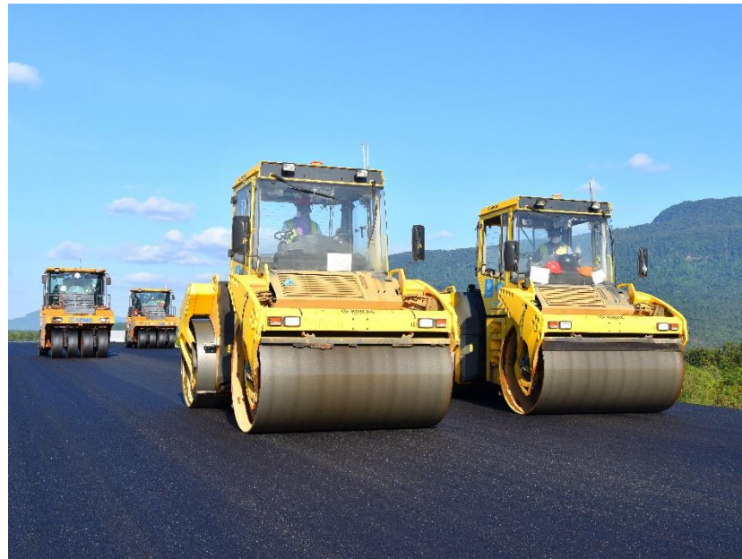
Figure 21. Compaction work site.
