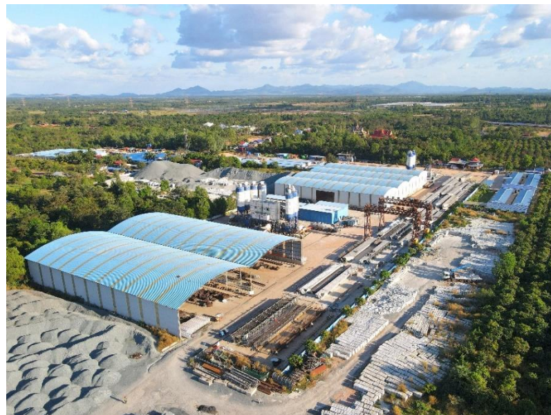
Figure 14. Mixing construction site.
