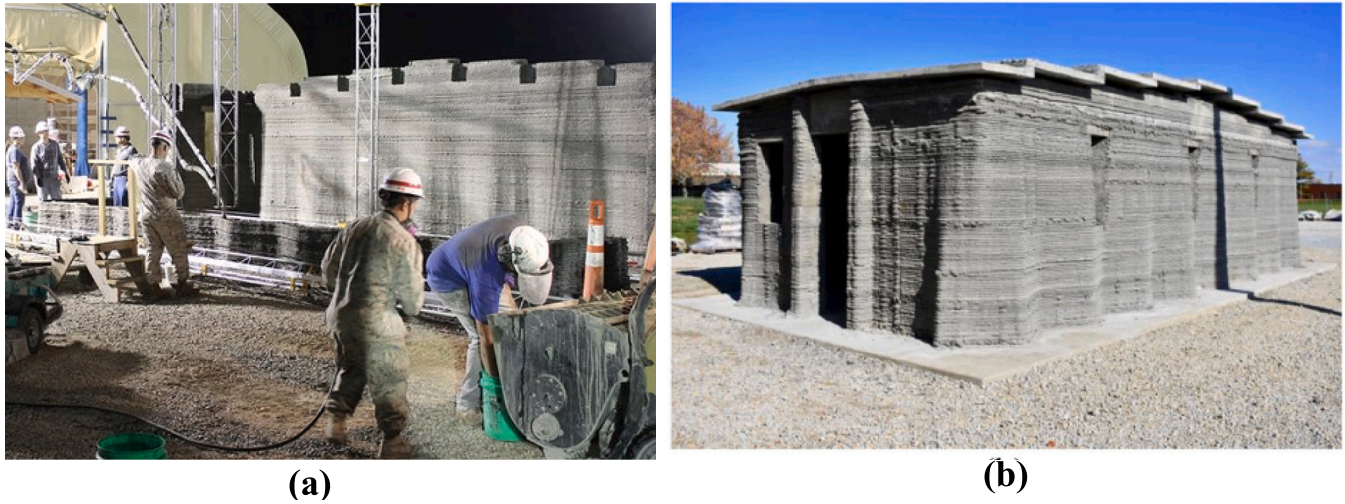
Fig. 8. ACES military project: (a) Printing process, and (b) completed structure [18,150] (Images have been declared public information by Marine Corps Website of US government and is not subject to copyright protection in the United States).
