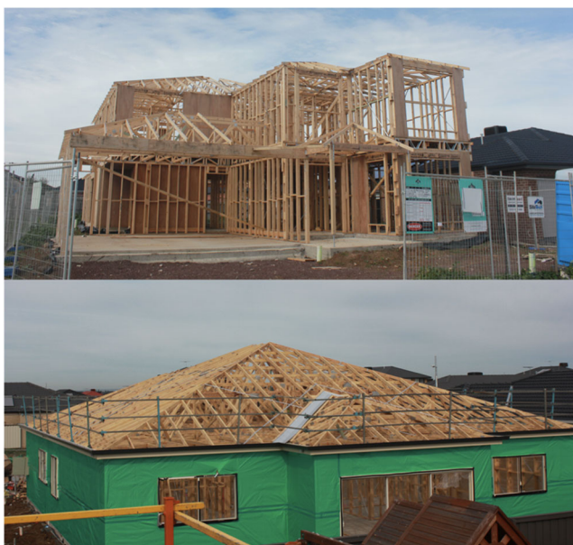
FIGURE 6 Typical timber-framed house construction in Australia.
