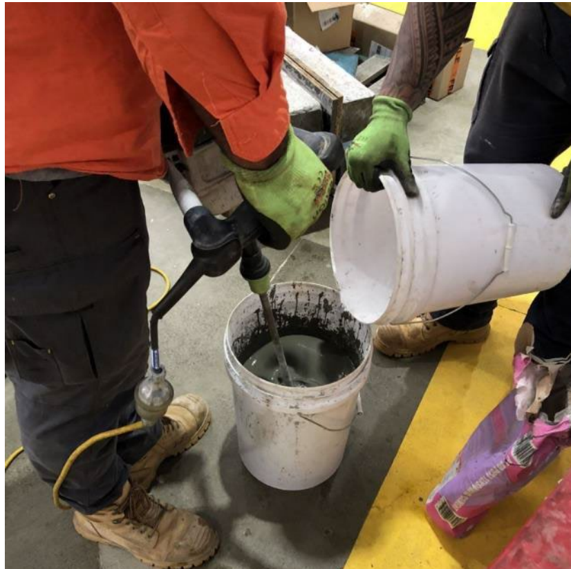
Figure 5.51 Mixing high-strength post-tensioning cement.
