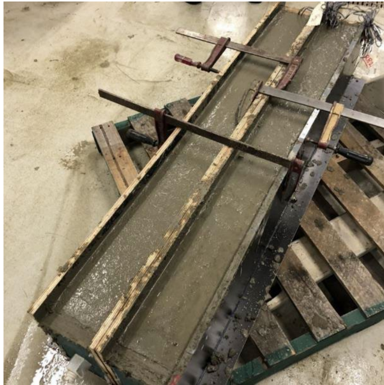
Figure 5.40 Placement of concrete.
