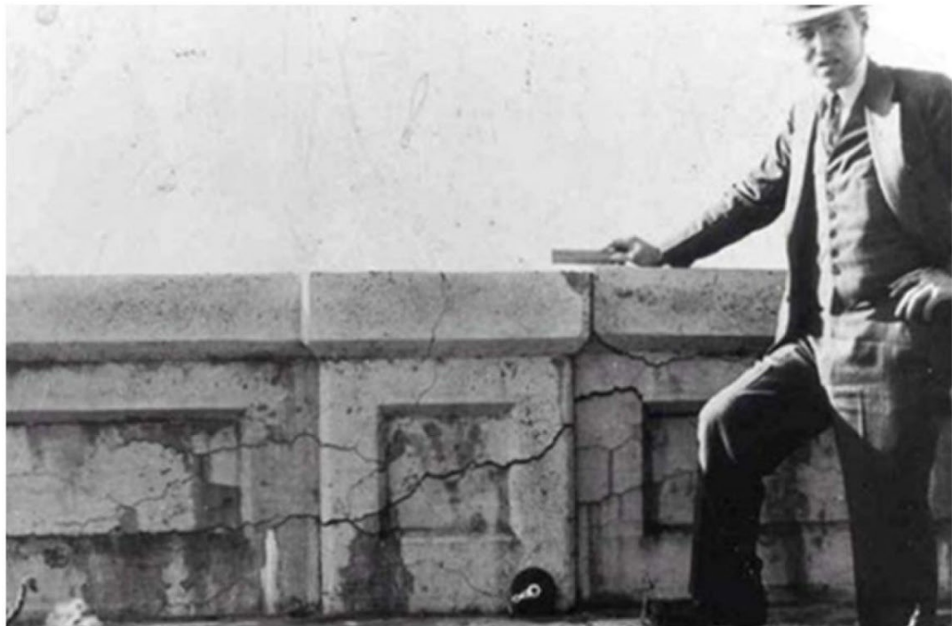
Figure 2.1 A bridge parapet wall with signs of Alkali-Silica Reaction damage captured by Stanton. (Adopted from Thomas and Fournier et al. 2013).
