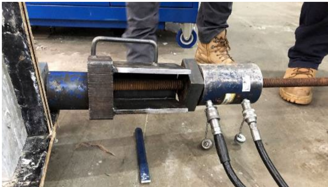
Figure 5.46 Setting up hydraulic jack for post-tensioning operation.
