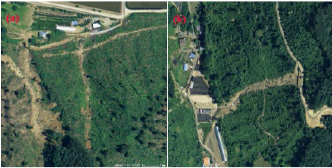
Fig. 2. Landslide damage on July 16, 2018.
