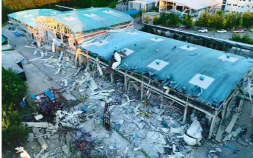
Figure 2 Hydrogen explosion accident in South Korea on May 2019, six casualties and several surrounding buildings (up to 100 m away) were seriously damaged [12]
