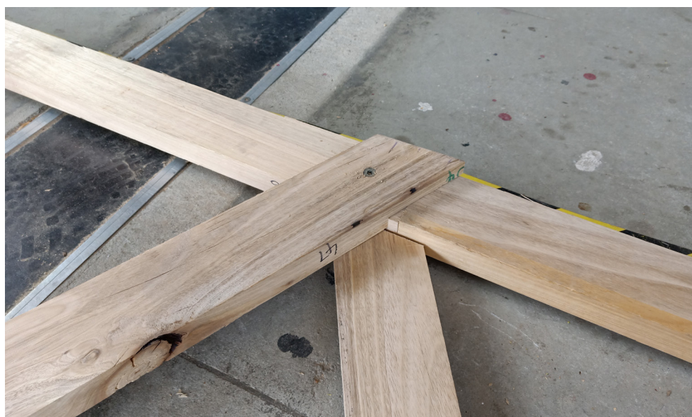
Figure 5.50 Alternate fixing method at intersection nodes
