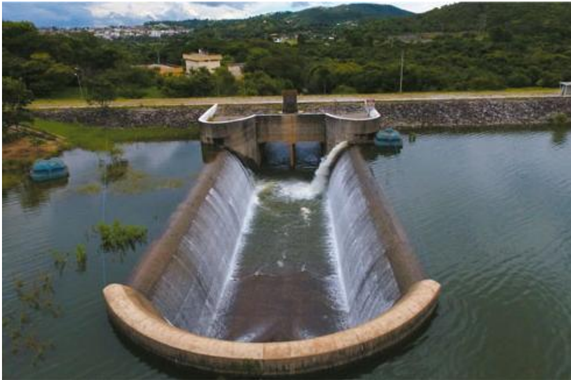
Figure 3.13 – Overflow in the spillway of Vargem das Flores reservoir, with pump installed in the right corner of the weir (31/01/2020)
