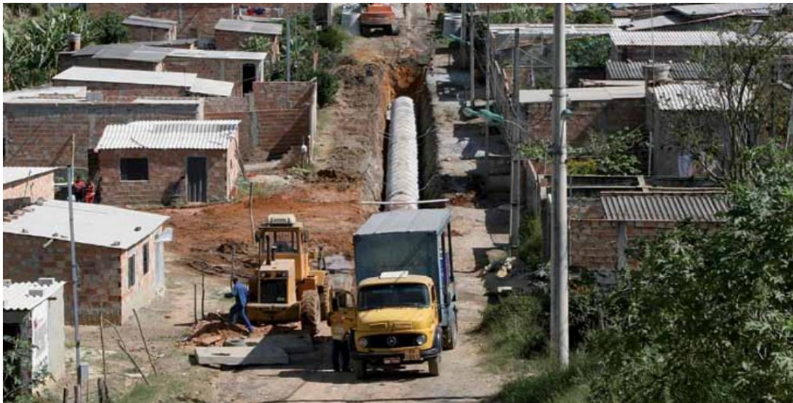
Figure 3.5 – Construction of sewage network in the region of Nova Contagem (2010)
