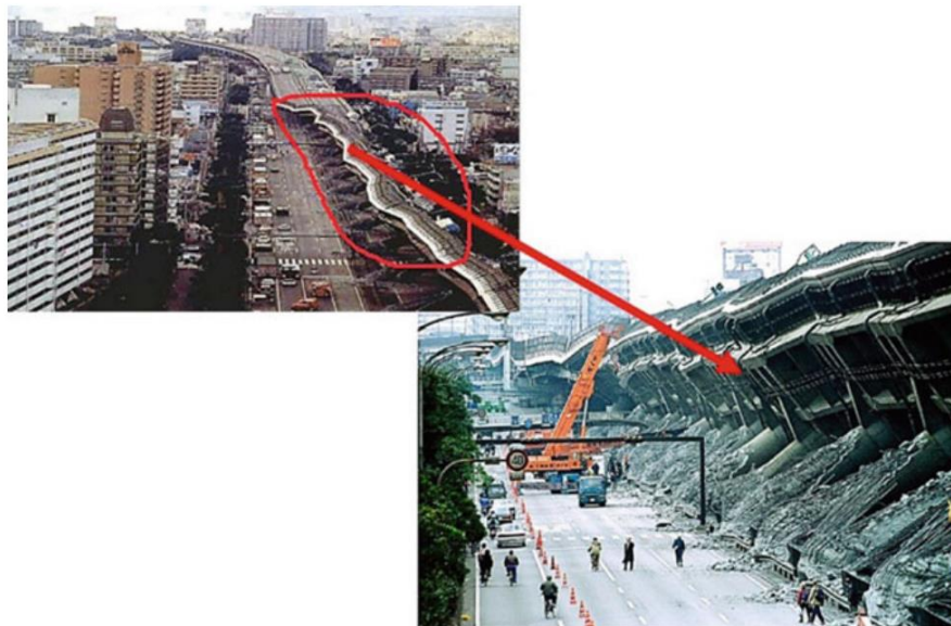
Figure 1.2 Hanshin Expressway collapse during Kobe Earthquake, 1995 (after Mylonakis and Gazetas 2000)
