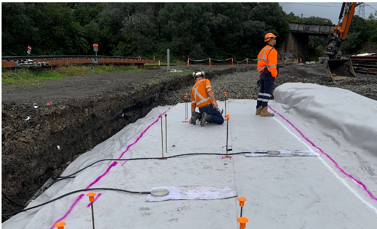
Fig. 9. Arranging pressure cells at the ballast-capping interface.
