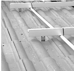
Figure 4.10 Rails Aligned on a Roof
