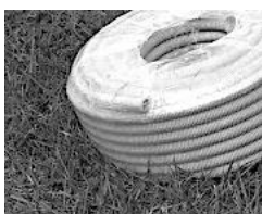
Figure 4.9 A Roll of Electrical Conduit Being Prepared for Installation
