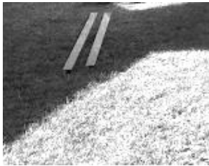
Figure 4.13 Two Rails Being Prepared Before Installation
