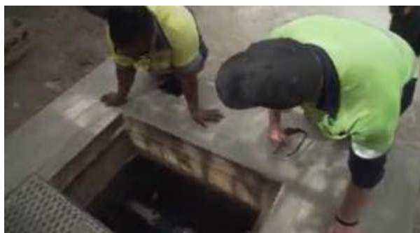
Figure 28. Partners working together to inspect wastewater systems
