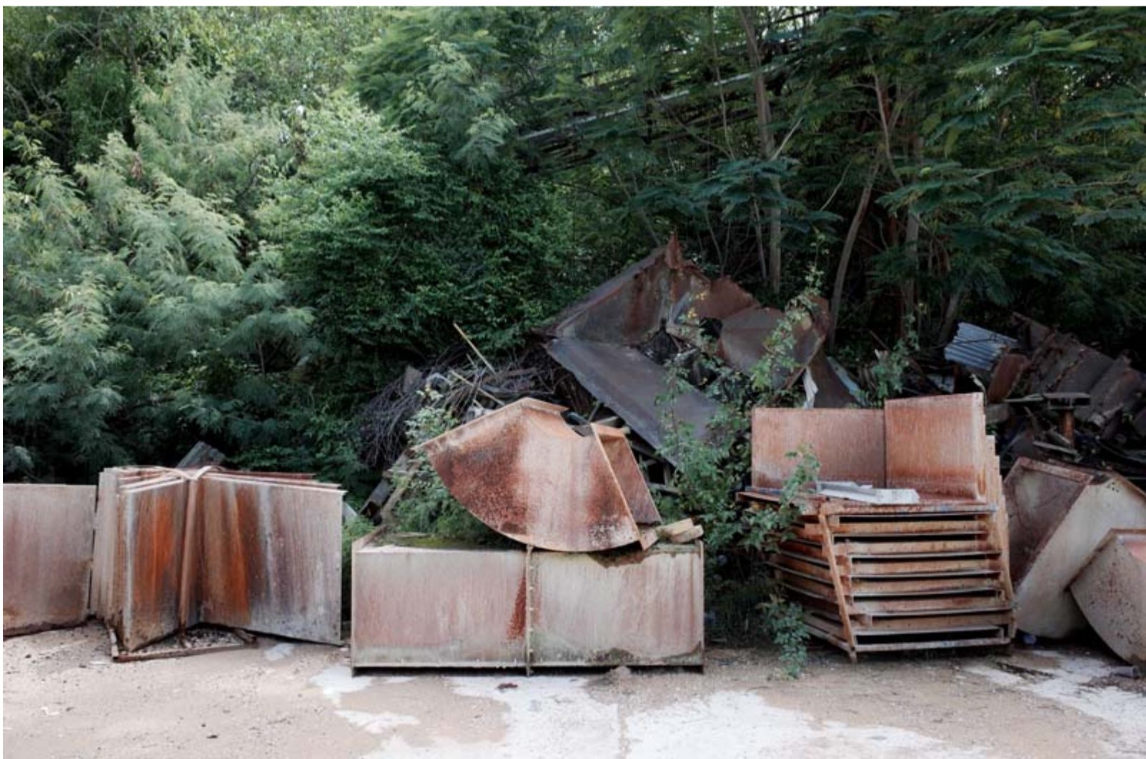
Fig. 26. More parts—ducts, hoppers, trays and roof sheeting—in front of a disused phosphate conveyor belt overgrown by the resurgent tropical scrub.
