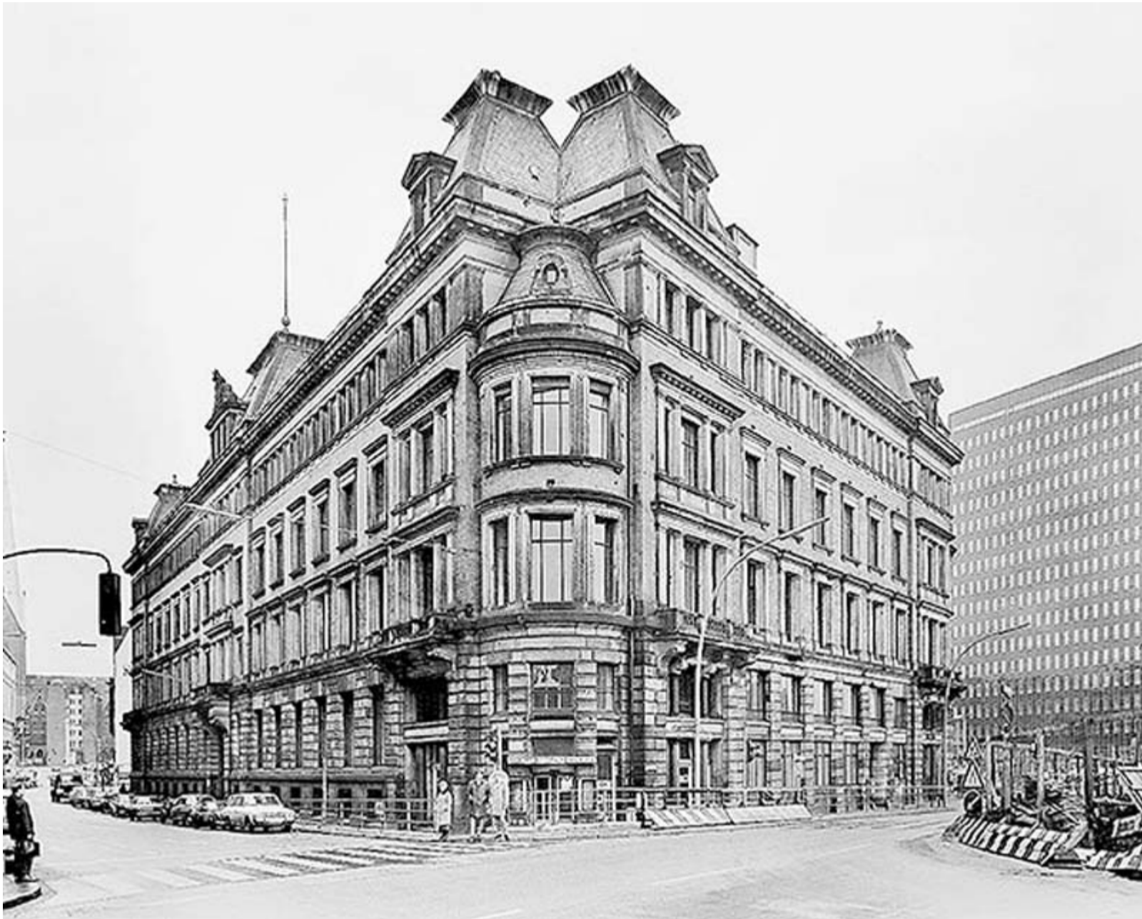
Fig. 8. The Dovenhof . Source: Commons.
