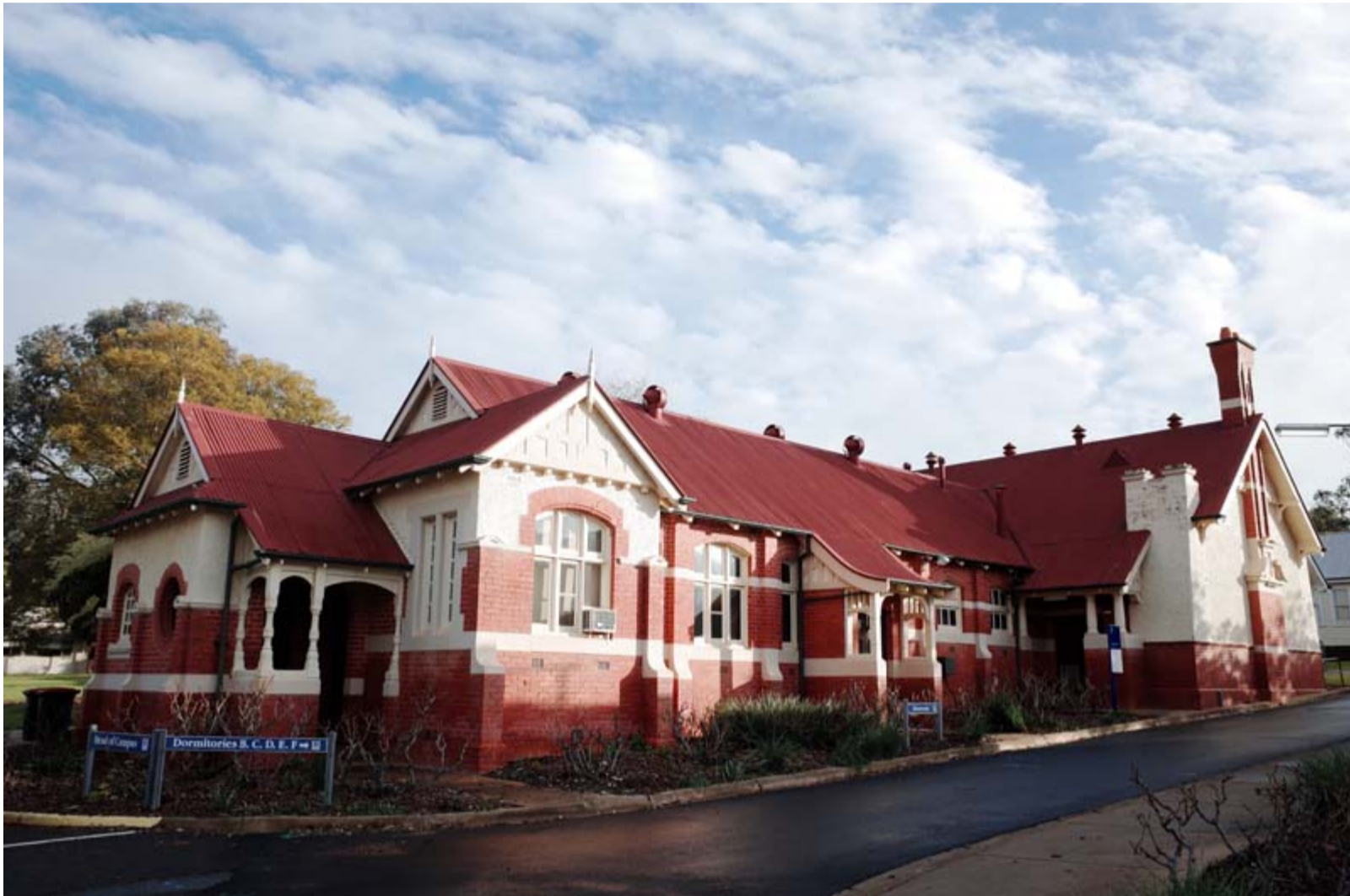
Fig. 17. Dookie College administration building and museum, formerly the college laboratory.
