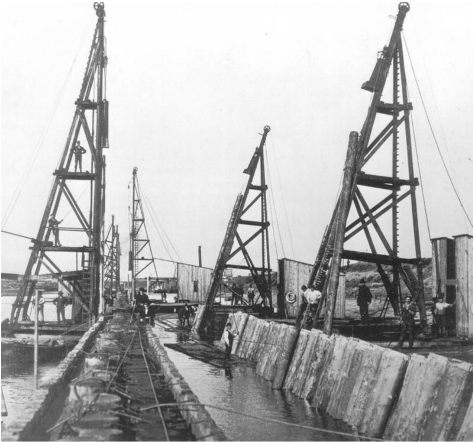
Fig. 36. Pile driving works at the Weserkorrektion , c.1889. Source: Commons.
