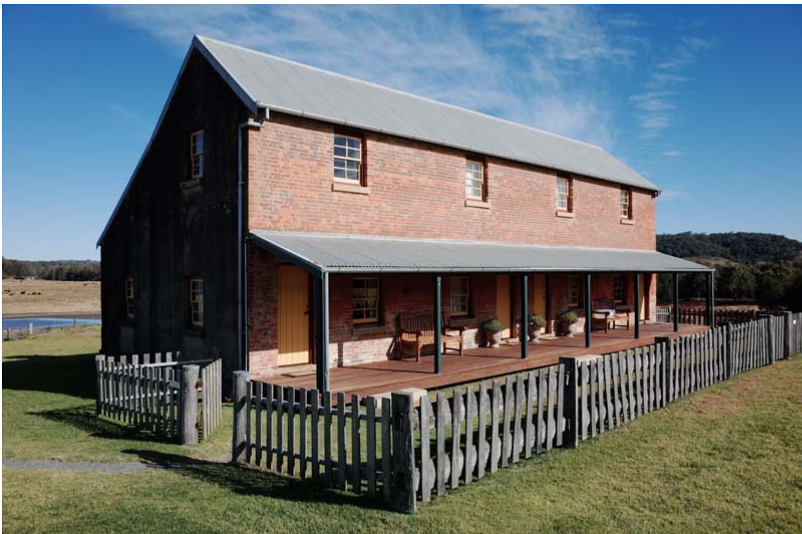
Fig. 6. The barracks built to house Tocal's 35 convict laborers during its development in the 1830s.
