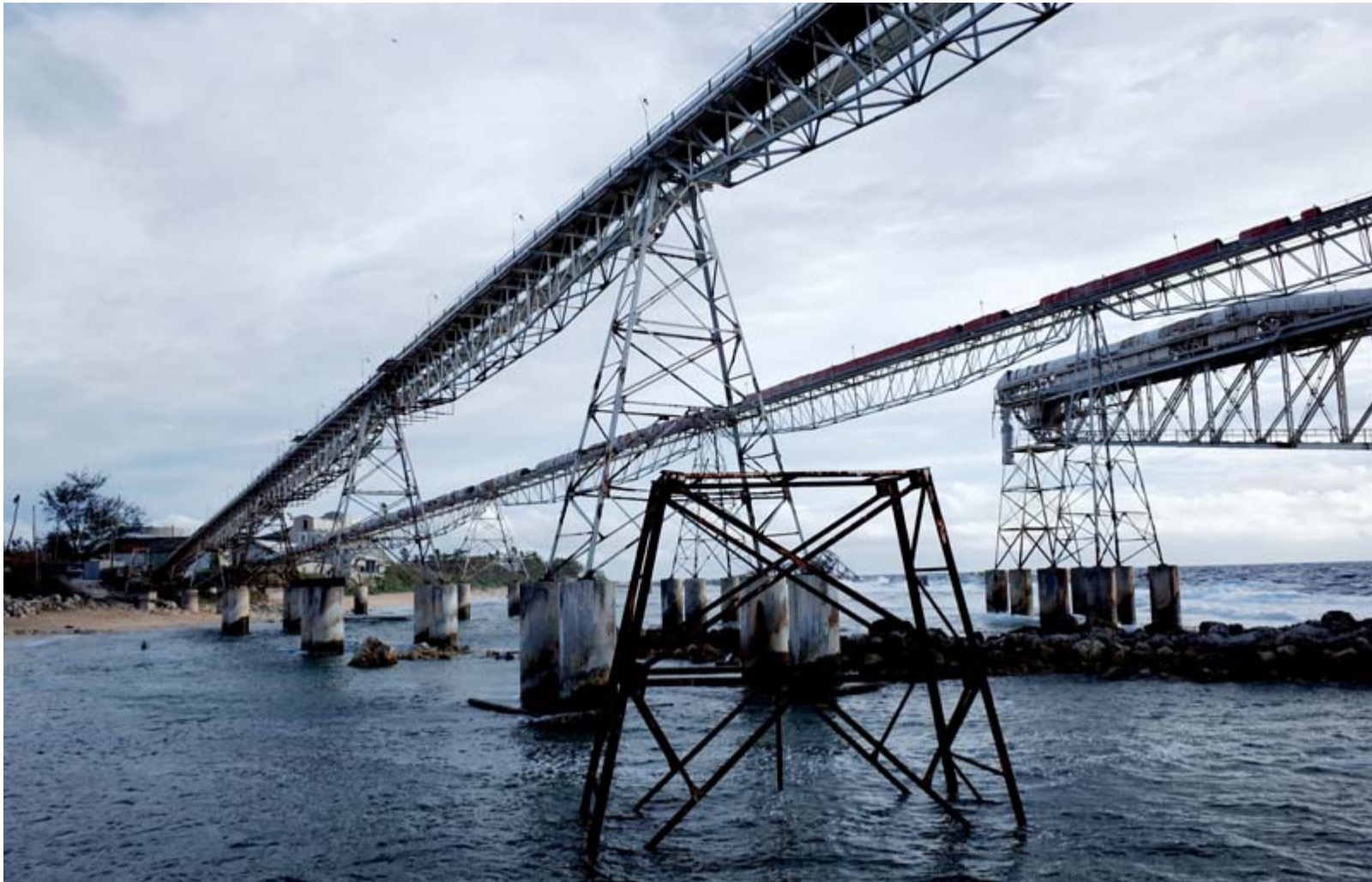
Fig. 18. Conveyors transport the crushed and dried phosphate to the cantilevers for loading.
