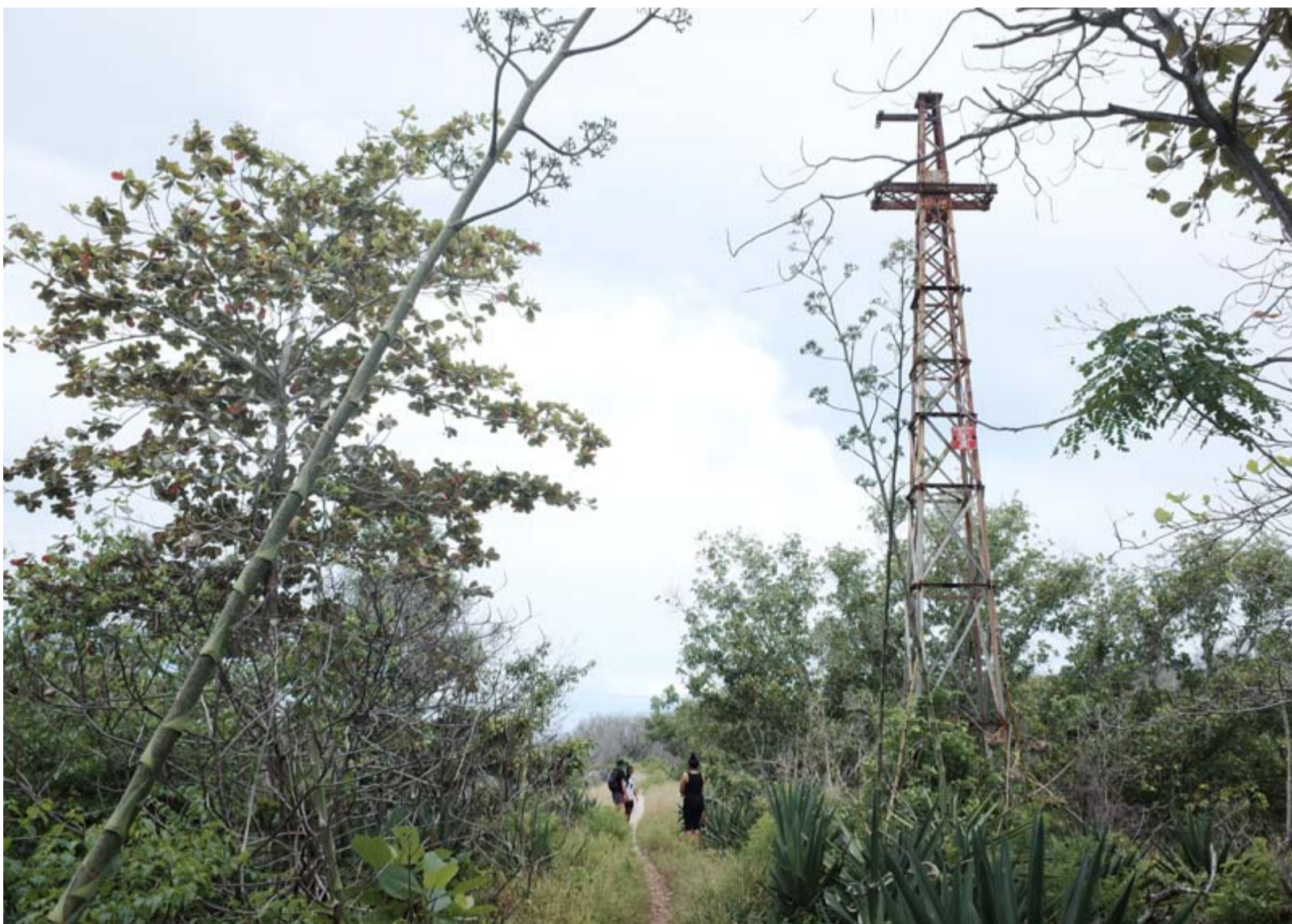
Fig. 29. One of the steel structures lining the main embankment at Topside, likely the base for the aerial cableway designed by the engineers J. M. and H. E. Coane of Melbourne.
