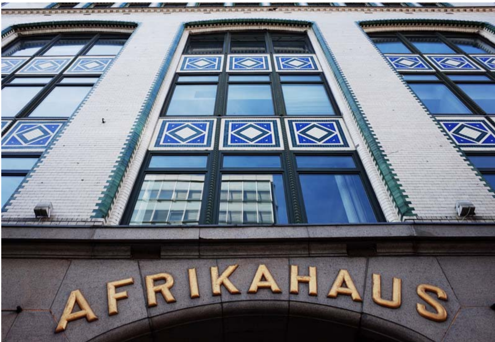
Fig. 11. The glazed masonry façade of the Martin Haller-designed Afrikahaus .
