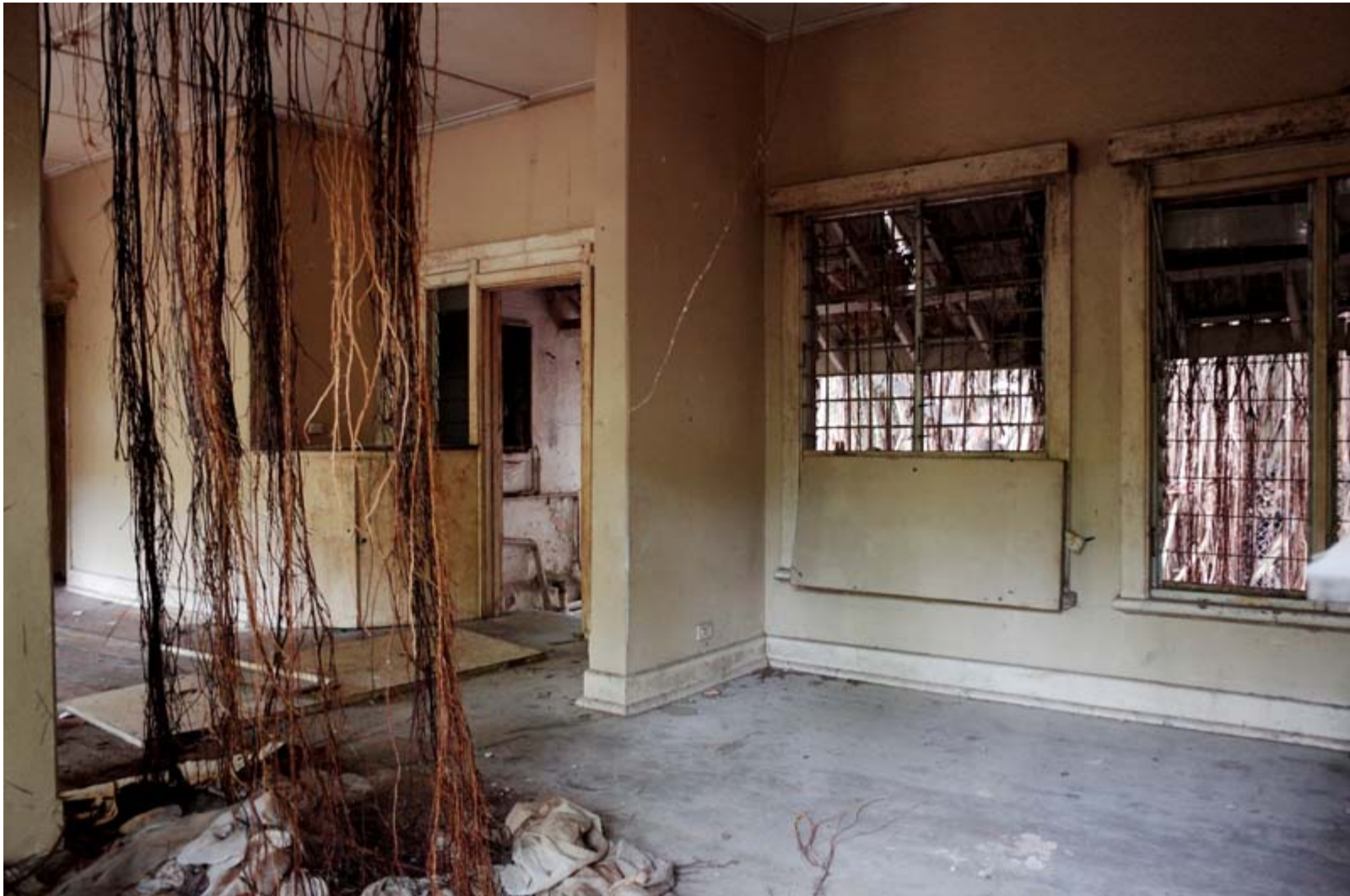
Fig. 32. The house is being slowly consumed by a large Banyan fig, its roots penetrating the asbestos roof and timber floor.
