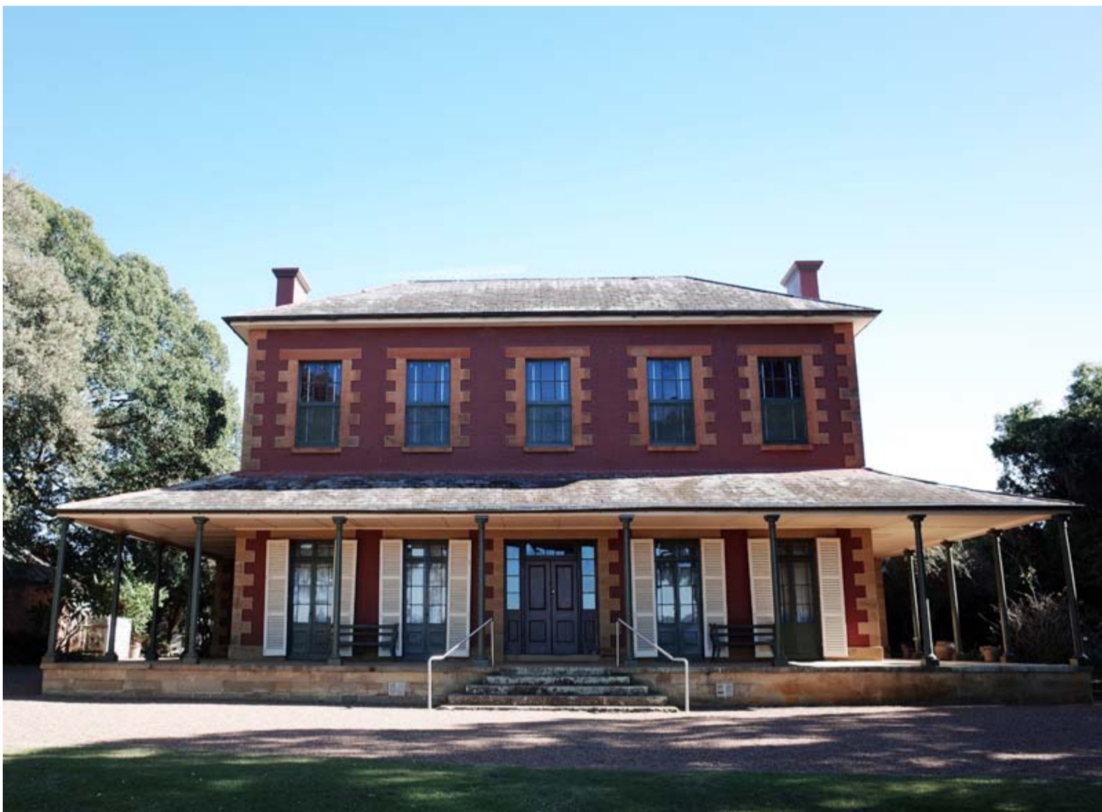
Fig. 7. Tocal Homestead was built to the 1841 design of the Scottish architect William Moir. It was constructed from sandstone with a slate roof, most of which was quarried directly from the Tocal site.
