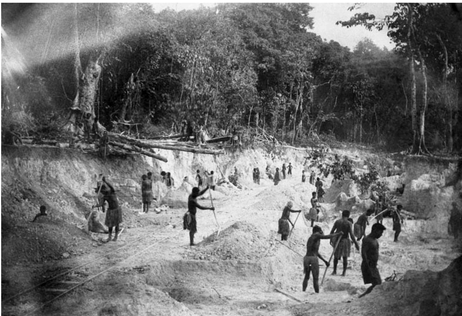
Fig. 24 – Indentured Caroline Islander laborers mining phosphate on Angaur using hand tools, c.1909. A tramway runs through the pit, connecting the mine to the processing facilities on the coast. Source: Deutsches Bundesarchiv, Sammlung Heinrich Hagedorn, Bild 223-153.
