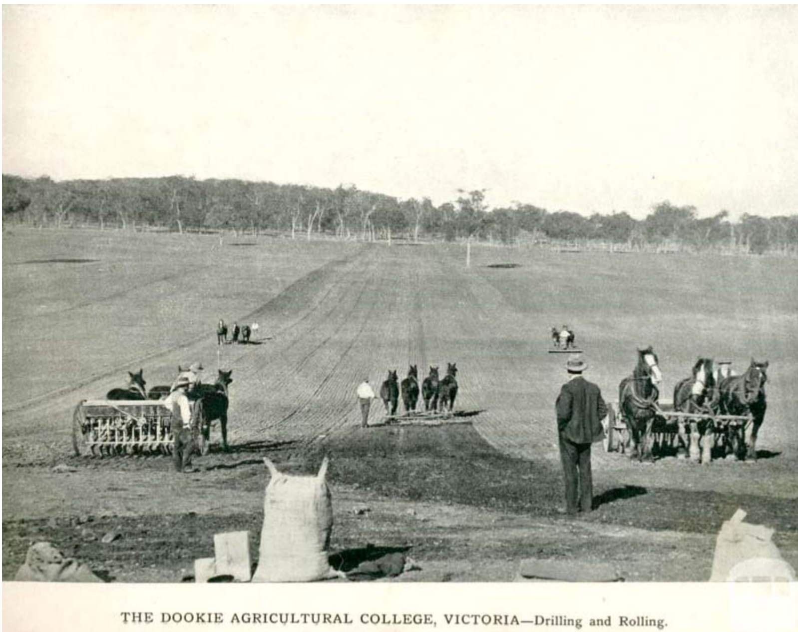
Fig. 22. "The Dookie Agricultural College - Drilling and Rolling." Drilling typically involved so-called "combines," which deposited both seeds and superphosphate in furrows at regular intervals and set depths. Source: Victorian Places.
