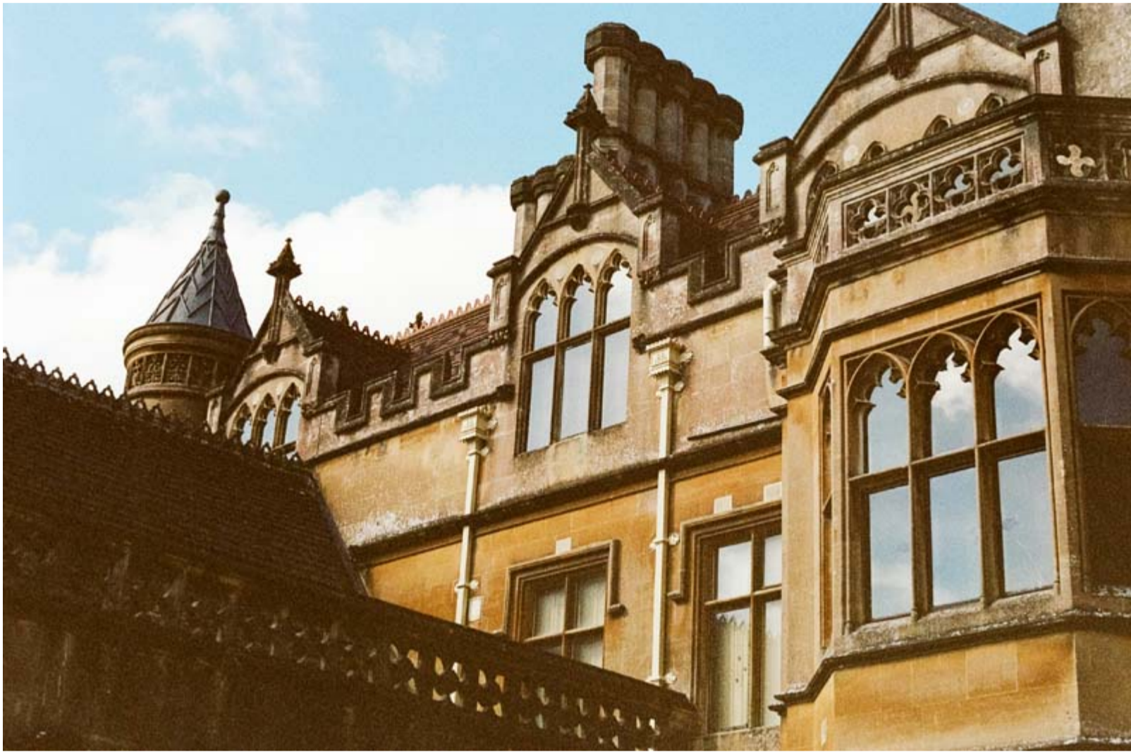
Fig. 12. Further additions made once Tynestfield House was inherited by William’s son, Antony, are visible in the colour difference in the stone.
