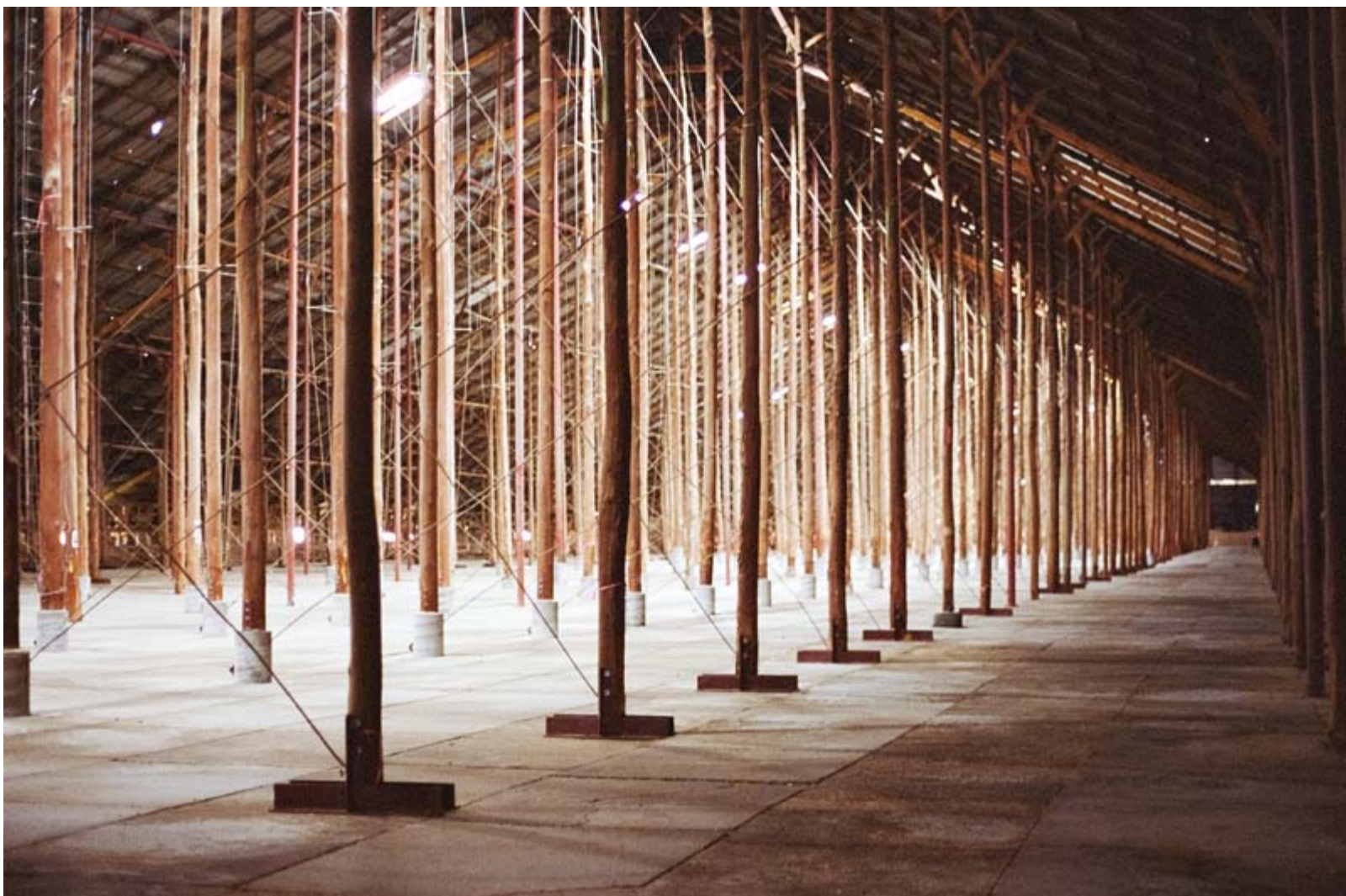
Fig. 32. A longer exposure photo of the Stick Shed's interior. The ties that cross-brace the tall poles wobble with each gust of wind that hits the exterior of the building.
