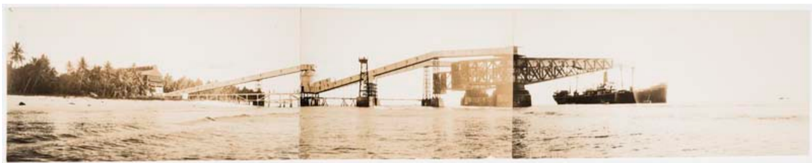
Fig. 19. The steel cantilevers and conveyor system used on Nauru in c.1932, during the period of the British Phosphate Commission. Maslyn Williams Nauru Photographs, State Library of New South Wales, PXB 293, Image 116.
