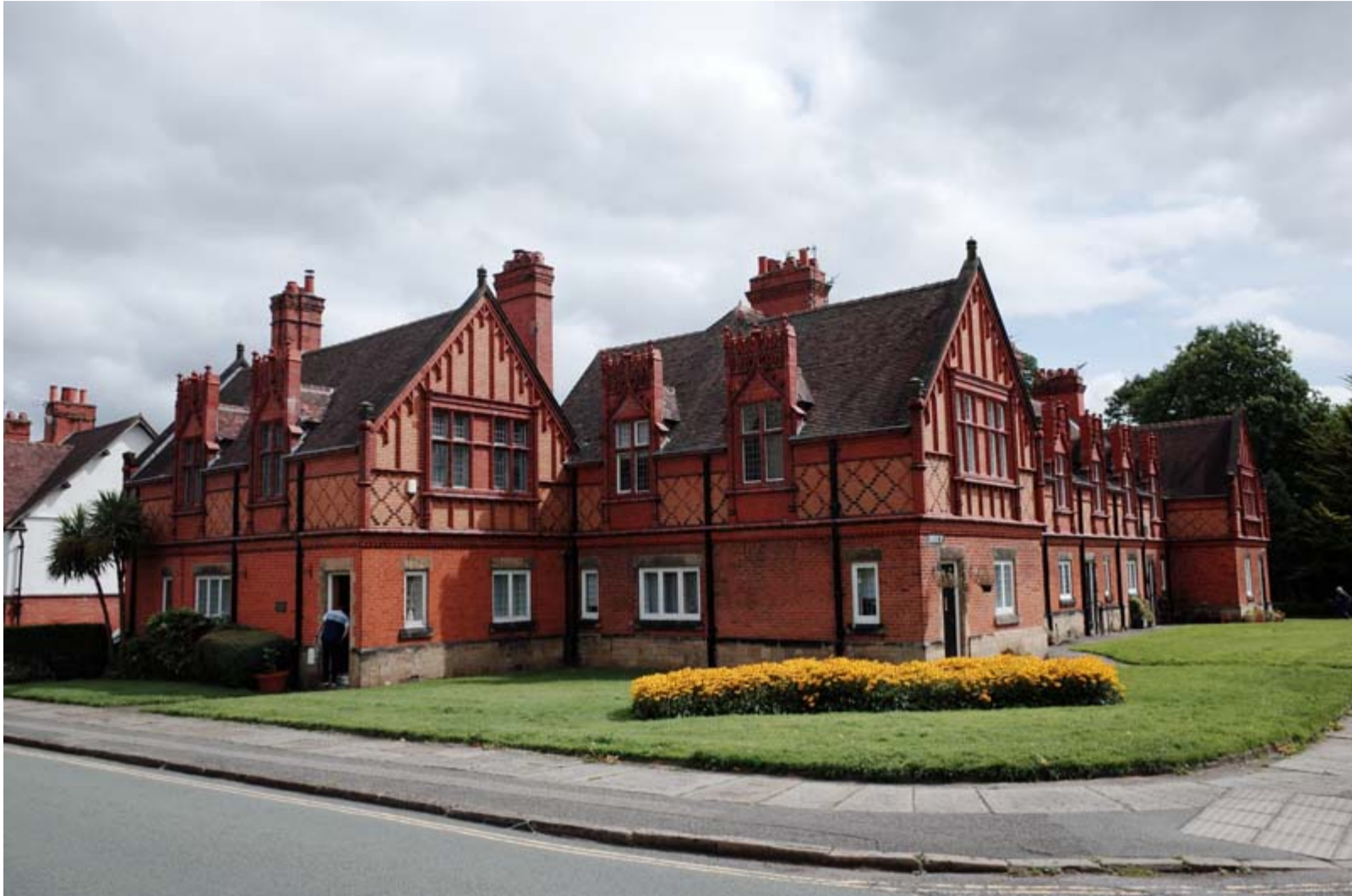
Fig. 29. Flemish brickwork was also popular for the housing in Port Sunlight.
