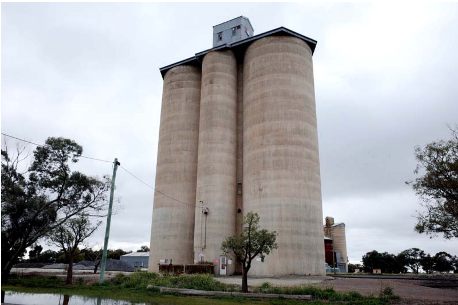
Fig. 28. Concrete wheat silos in Warracknabeal built in the 1930s, now redundant as grain growing has diversified.
