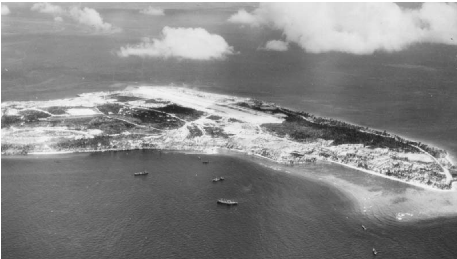
Fig. 25 – Aerial view of Angaur from the west. Apart from the airstrip, located at the top of the image, the white areas indicate phosphate mining sites. The major mines on the island are visible to the left of the image. A string of strip mines runs along the length of the runway. Source: US National Archives, Caroline Islands, 1944, 204969950.
