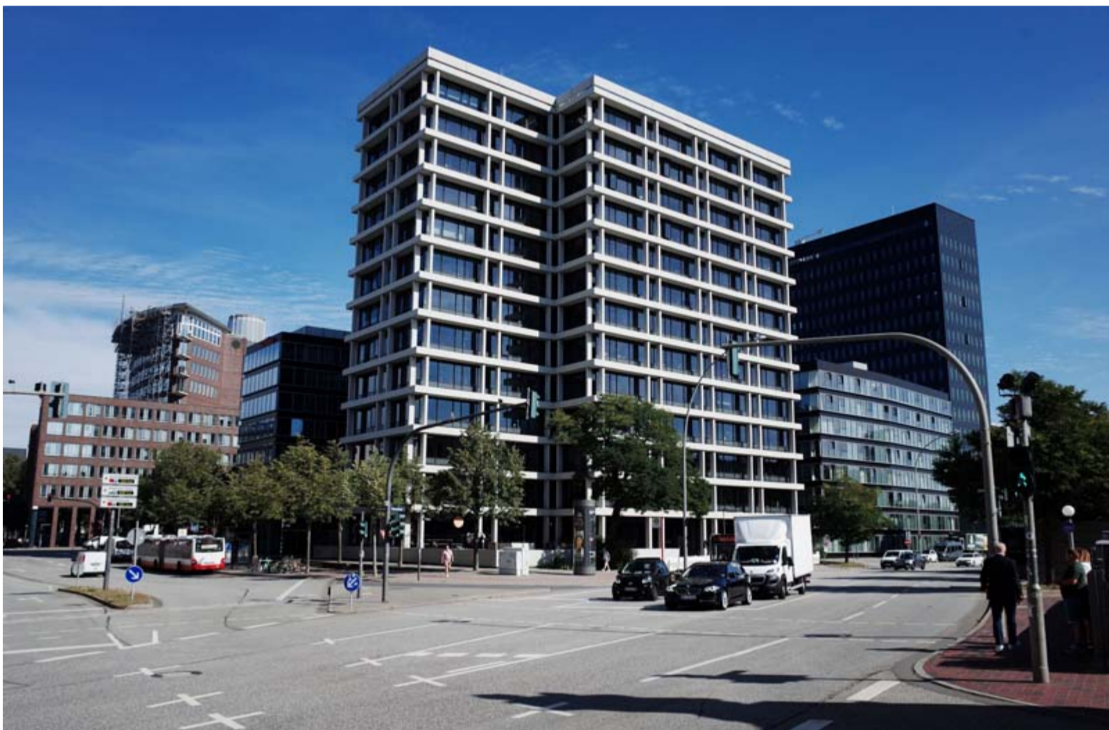
Fig. 10. The Dovenhof was demolished in 1967 to make way for the former headquarters of the newspaper Der Spiegel .
