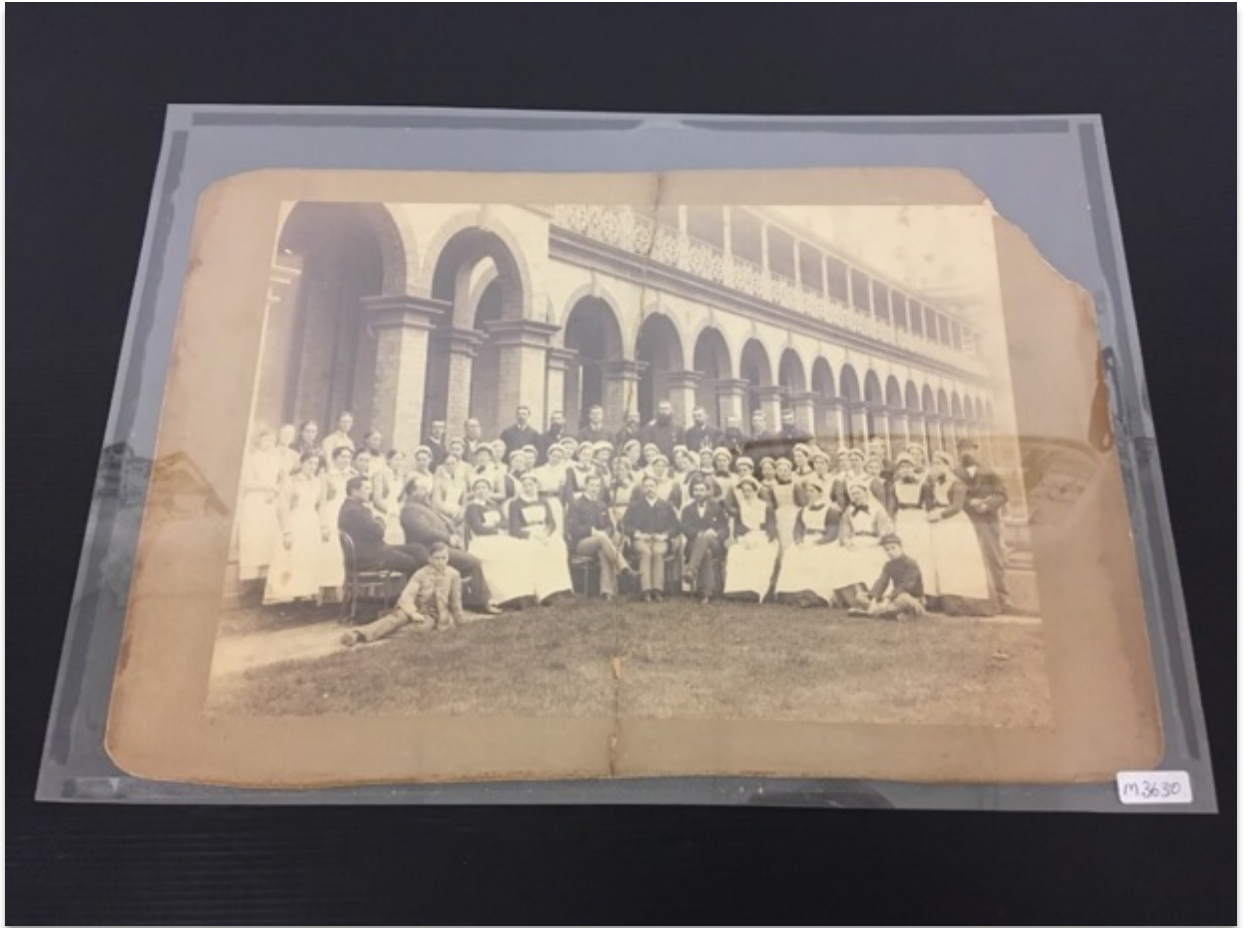
Original print of showing rear view of RPA, 'All Staff', c. 1885, 240mm high x 360mm wide Source: Scott Andrews, original photographer unknown
