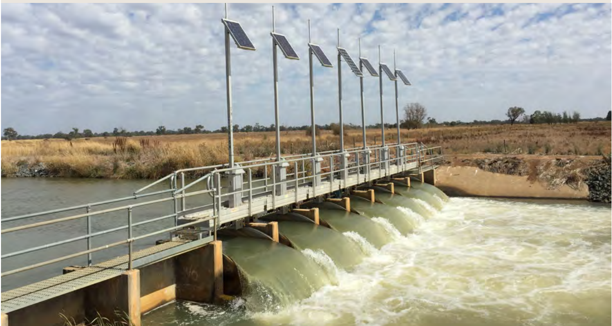
Multibay flumegate regulator, Macalister Irrigation District (credit: Southern Rural Water)
