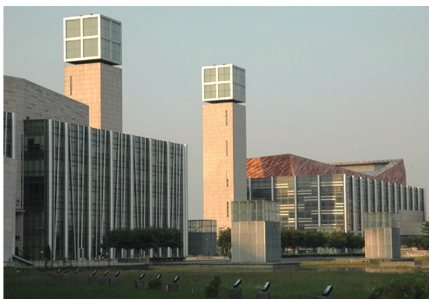
Figure 7. Shunde Library left and Shunde Performing Arts Center, 2005. Source: Photo by the author
