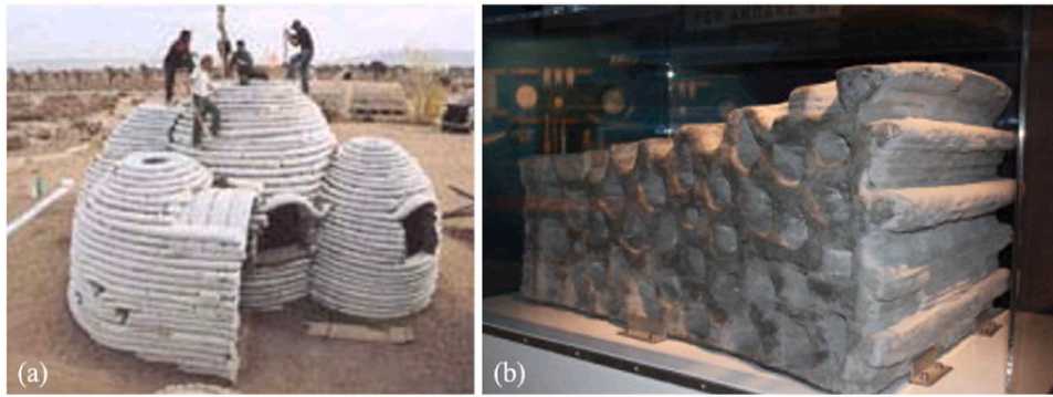
Fig. 34. (a) Contour Crafting printed [207] and (b) D-shape printed lunar structures [204].
