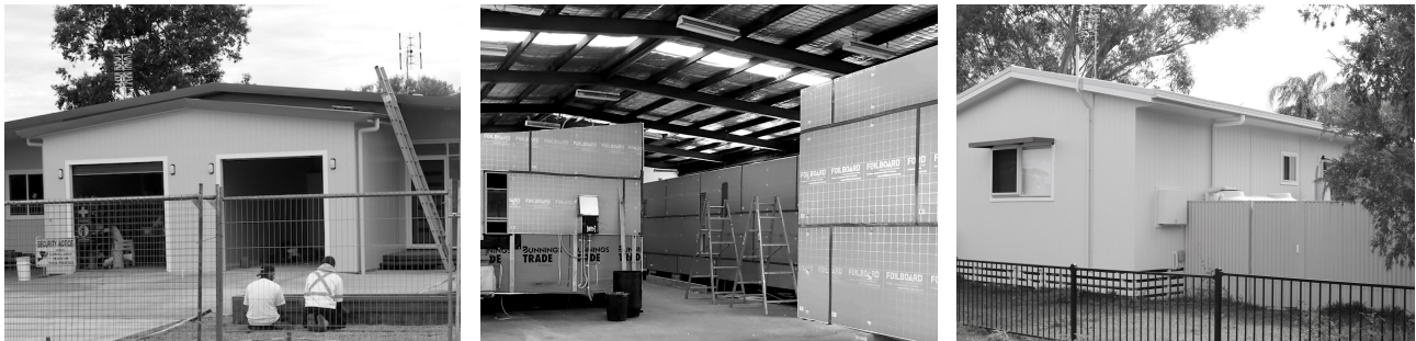
Figure 03. Photograph of SIP (left), GlueLam (middle), and Podular (right) construction for AHO Innovation Program in Moree. From Photographs by Campbell Drake, 2020
