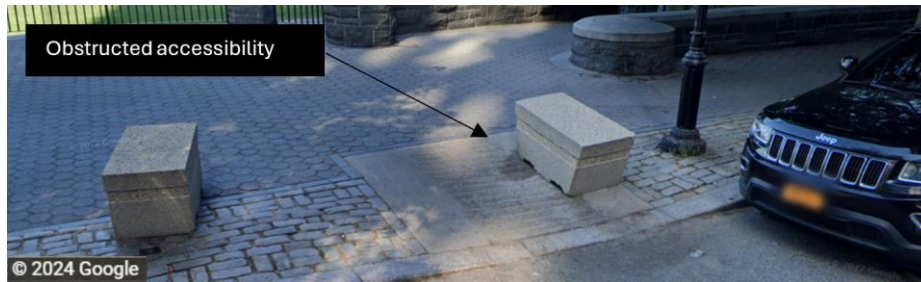
Fig. 2. Obstructed accessibility ramp post-protective security installation on River Terrace at Battery Park - June 2022. Source: Google Streetview and annotated by authors [26]
