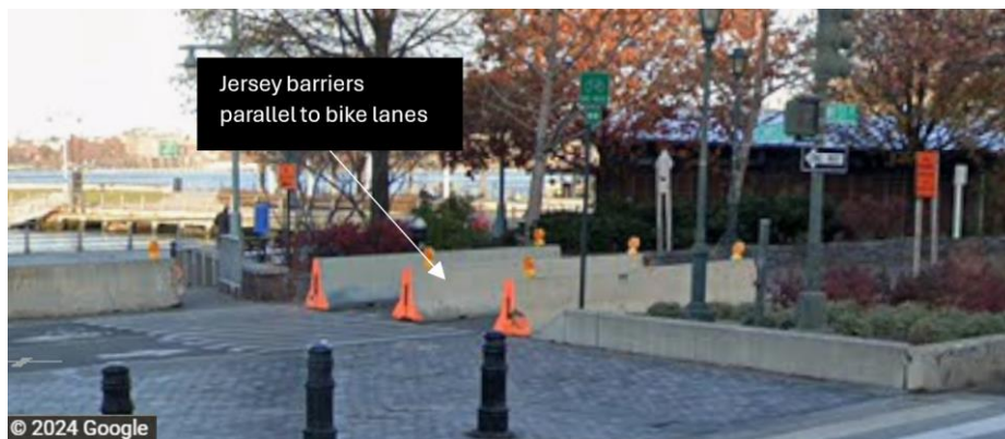
Fig. 5. Modified Jersey Barriers on Hudson River Greenway post-community consultation – June 2019 [36] Source: Google Streetview and annotated by authors
