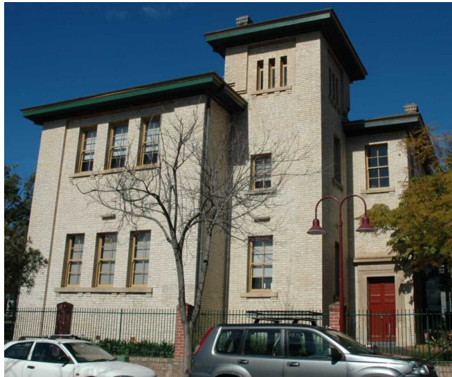
Figure 9: Milsons Point Public School designed by Kemp, 1887. Source: Kirsten Orr.
