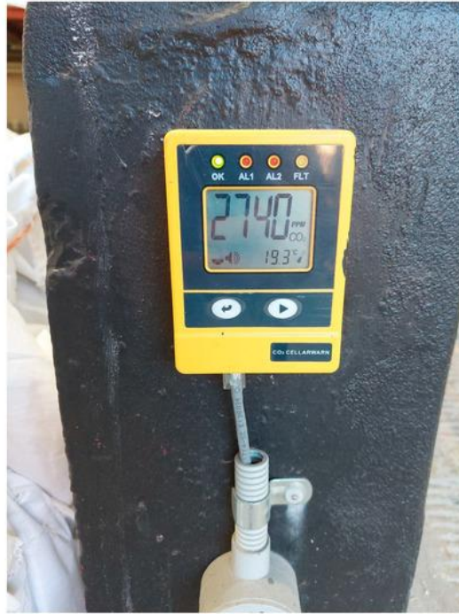
Figure 1. An example of a hard-wired CO 2 monitoring system used in an Australian brewery.
