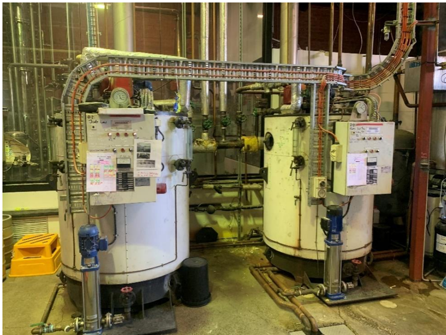
Figure 40. Two Simons 500 kW boilers within a working brewery.
