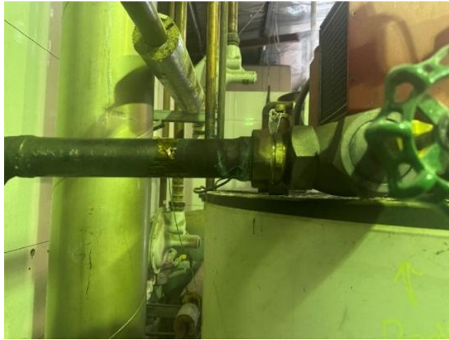
Figure 39. Hot pipe (dark pipe, running horizontally) used as the waste heat source within a working brewery.
