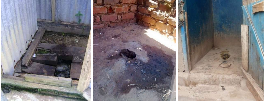
Figure 3.5 Unimproved (left and centre) and improved pit latrine with cleanable slab (right)
