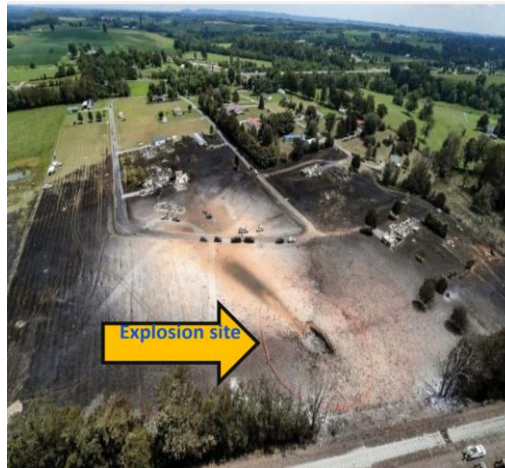
Figure 1.5 Burned area and explosion site in Lincoln County, Kentucky [30].
