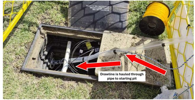
Figure 11: Field technicians successfully hauled drawline through conduits.
