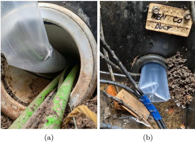
Figure 9: Examples of deployments in active nbn conduits of size (a) P100, and (b) P50.
