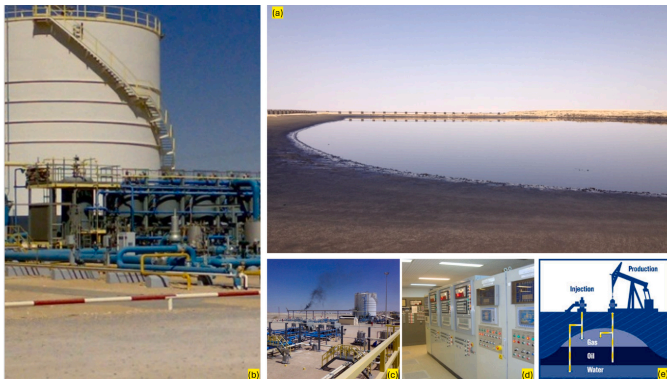
Fig. 5. Water injection system of oily wastewater HOO-Libya(a,b, c and d); Water injection system (e) (Engineering, 2016).
