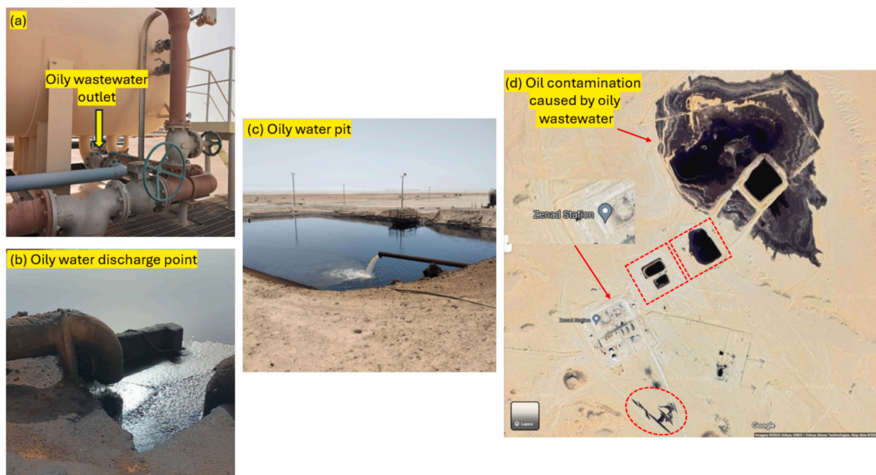
Fig. 4. Oily wastewater a) outlet from the production separator, b) discharge point, c) water pit, and d) The Google map reveals significant oily wastewater contamination at the HOO-2024.
