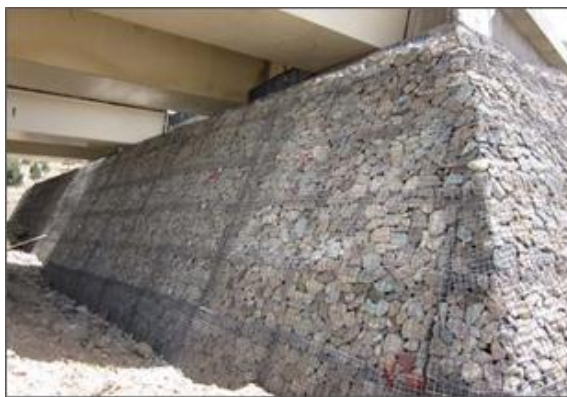
Figure 3. The view of the Milad GRS bridge abutment with gabion facing
