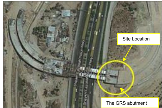
Figure 2. Completion of the bridge deck in 2011 (Courtesy of Google Map)
