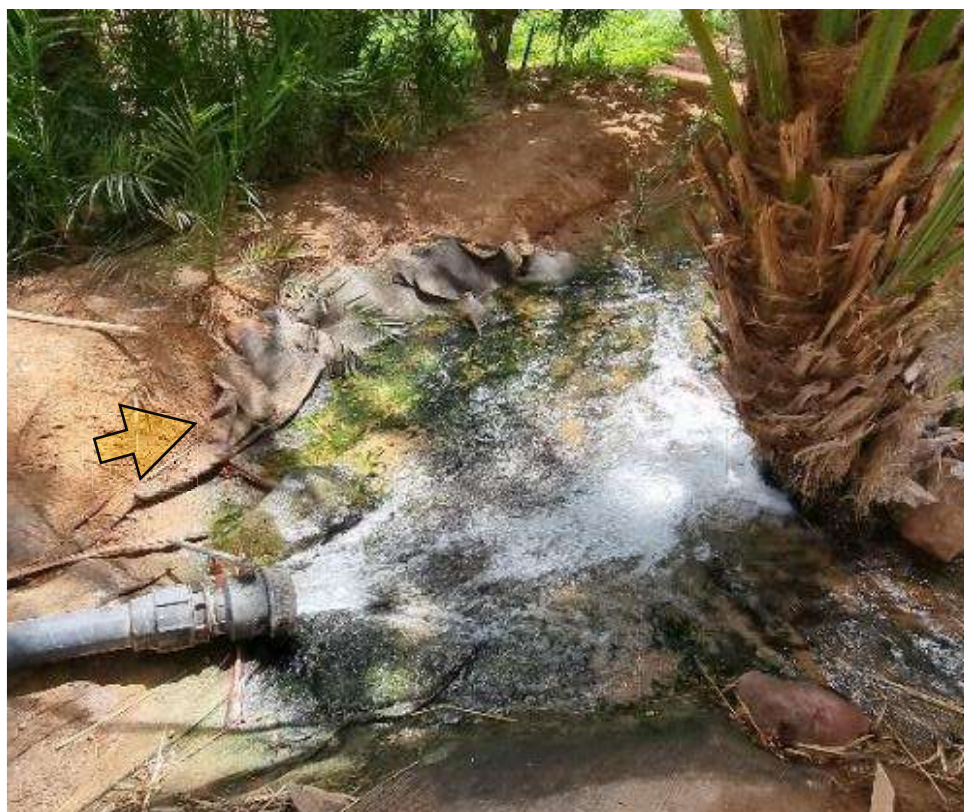
Figure 5-32: This is one of the places where a blanket is used to protect the soil from the strong water flow. Source: Photo by the researcher.
