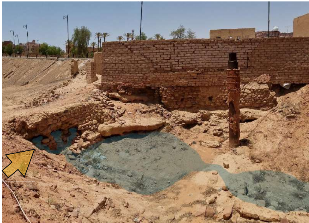
Figure 5-17: Top: The open part of the Shalal Spring. Many obstacles that may affect the water flow can be seen. Source: Photo by the researcher. Bottom: This photo shows the most famous water spring in AlUla, Ain Tadeul (Tadeul Water Spring), highlighting the soil collapse at its exit. Source: Photo and modification by the researcher.
