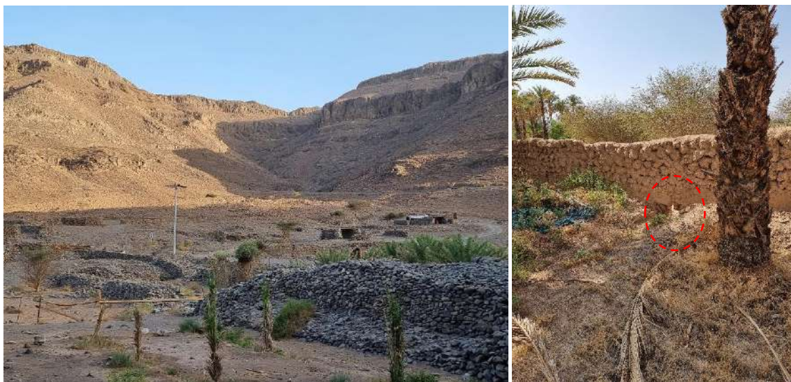
Figure 5-22: The left photo shows a wall made of rocks. The right photo shows a wall made of clay bricks and shows how water can still access the oasis. Source: Photos by the researcher.
