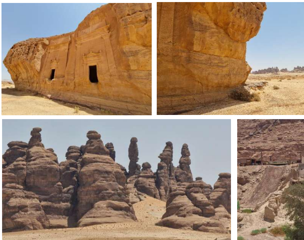
Figure 6-13: Photos showing the erosion occurring at different sites. Source: Photos by the researcher.
