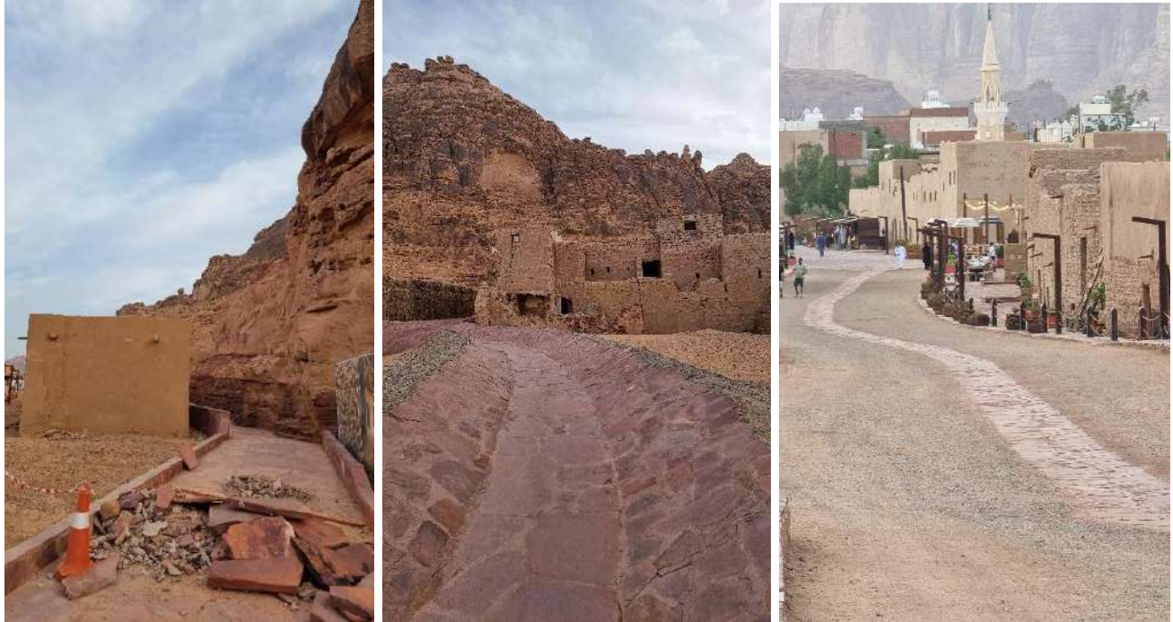
Photos 5-28: Left: the photo shows where elders used to implement rocky dams; however, the site has changed owing to the current development to make the site a tourist destination. Middle: The photo shows a new paved water canal collecting and redirecting water coming from the mountain. The traditional one was paved with soil, which allowed plants to grow and contributed to reducing the water speed; this one may increase the speed of the flow. Right: the photo shows another new water-harvesting/management technique that is not related to the local TEK of the community.
