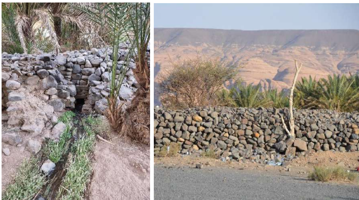
Figure 5-23: Elders noted that these walls allow the water to go into the farm gently by having small gaps between the rocks. This type is common in the Shalal area next to the volcanic mountains. Source: Photos by the researcher.
