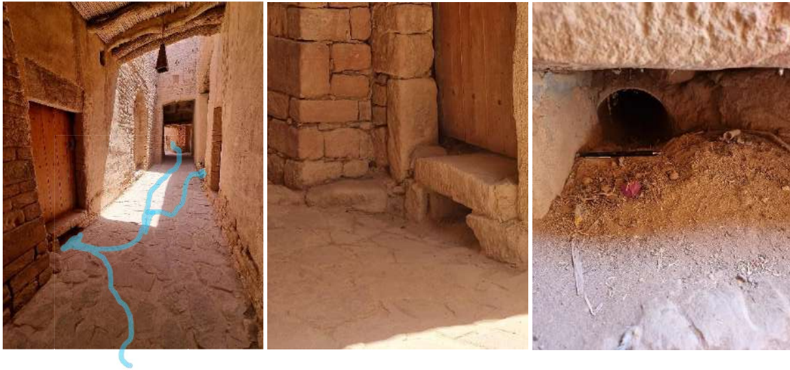
Figure 5-38: These photos show one of the water canals that harvests the rainwater coming from the mountains and redirects it to the oases. Source: Photos and modification by the researcher.
