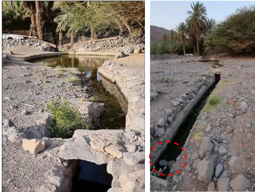
Figure 5-36: Left: the photo shows Al-Berkah , which collects water coming from the water spring, where I found one of the locals cleaning and removing rocks and algae. Right: the photo shows that, even when there is a barrier that protects the canal, there are still some fallen rocks inside, which disturb the flow. Source: Photo by the researcher.
