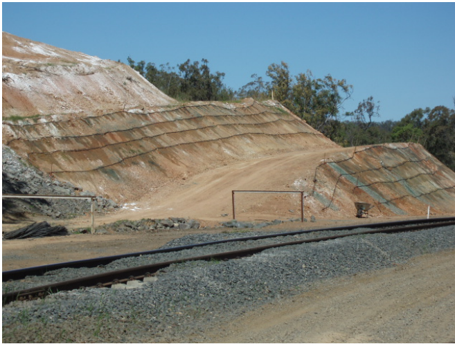
Figure 6. Holmes cutting site – lowest two batters showing emitter wetting fronts.
