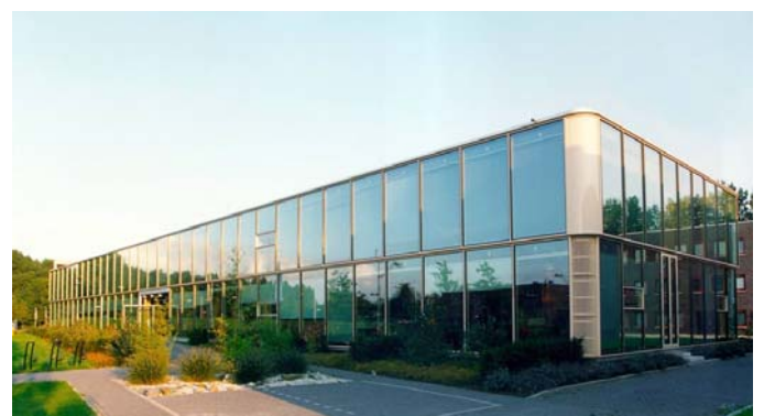
Fig. 2. The XX office building lasting for 20 years only. (Ref. 9)
