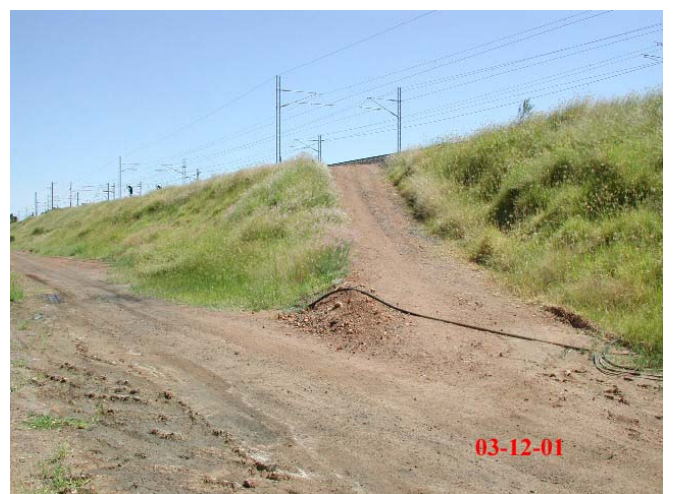
Figure 10. Riverside Mine site. Drip lines were laid on all batter sections at row spacing between 1 m and 2 m.
