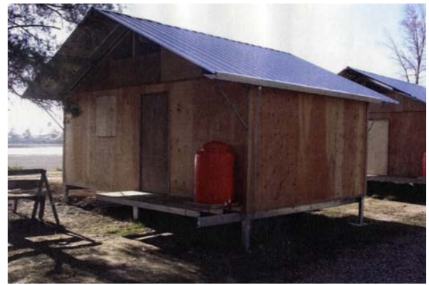
Fig. 4 Transitional shelter (Ref. 2)
