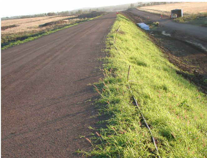
Figure 12. Bauhinia Site. Grasses established before track was laid. Three rows (1 m spacing) of drip lines were laid at the top batter section only.
