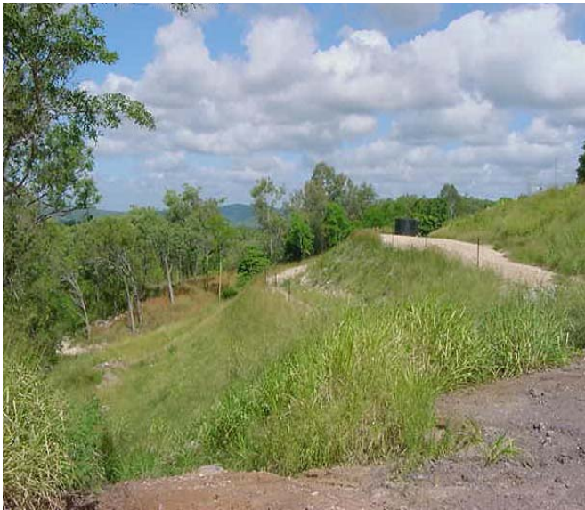
Figure 11. Black Mountain Derailment Site. Drip lines were laid on all batter sections at row spacing between 1 m and 2 m.
